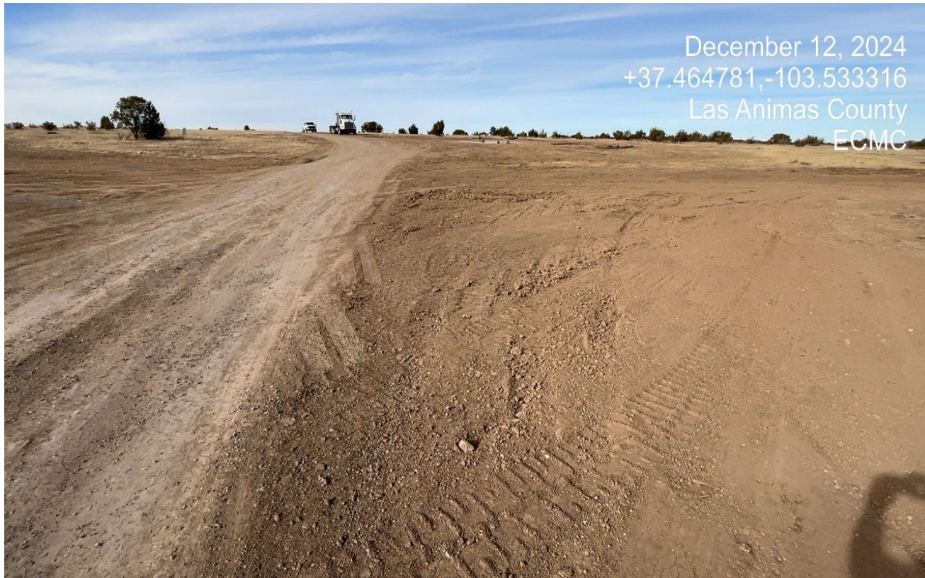
Photo 9. South side of the location facing north. The disturbed soils are not establishing vegetation. Vehicle use has compacted the top soils.
