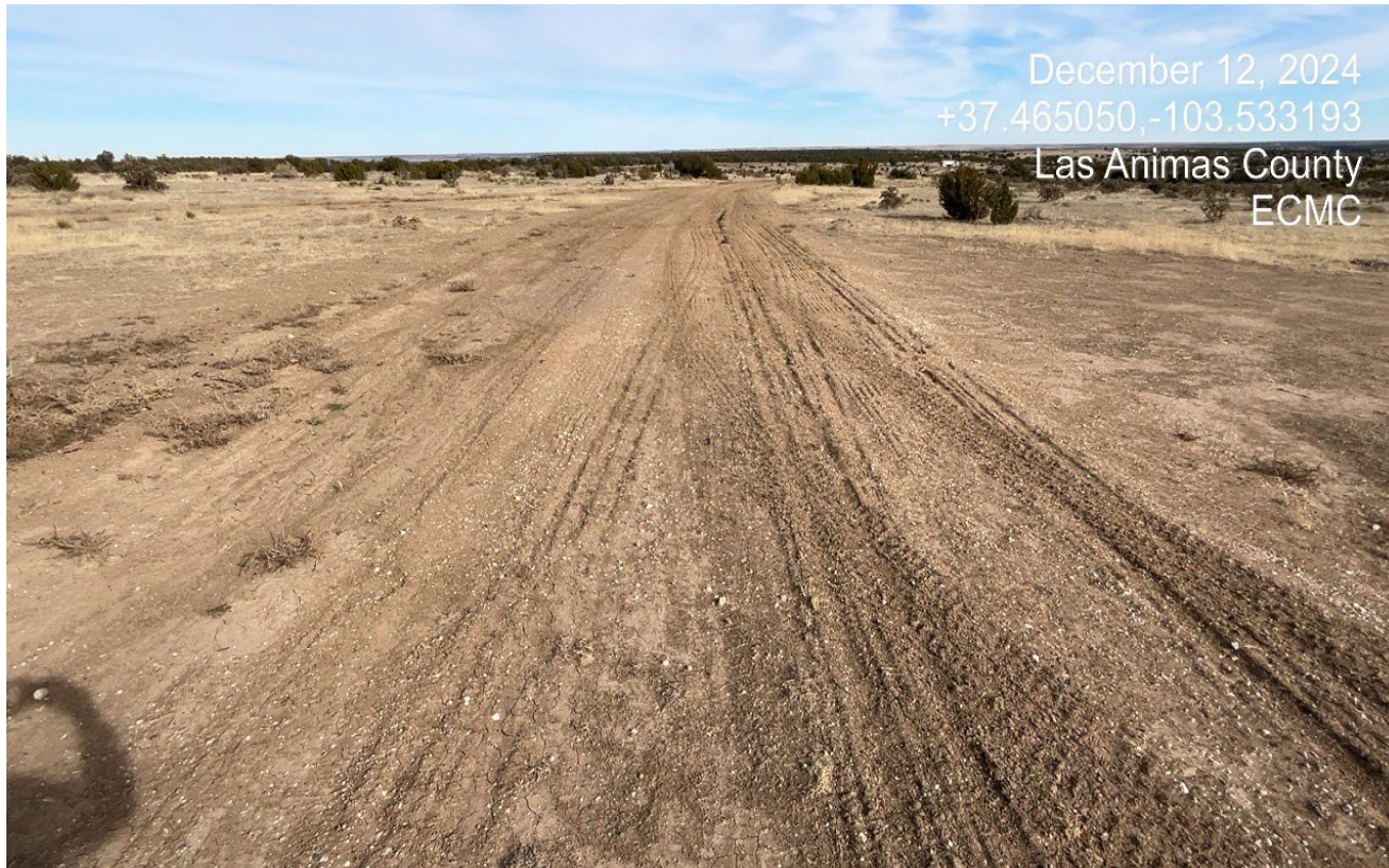
Photo 6. Facing east toward the flowline disturbance which has not established vegetation. Soils are not stabilized and are susceptible to erosion.
