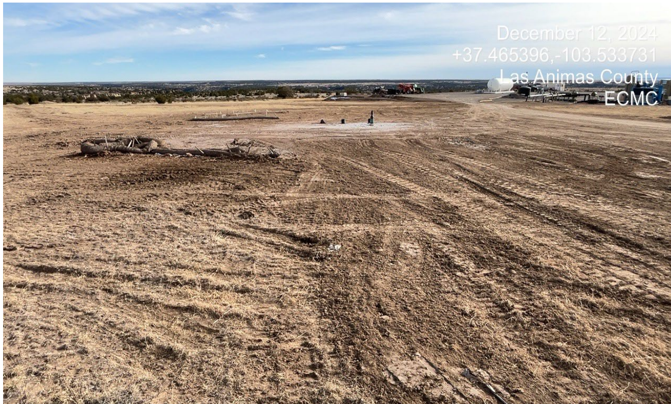
Photo 3. Facing southeast toward the wellsite. It appears recent work has been performed and the soils have been disturbed. The wattles are displaced and not maintained.
