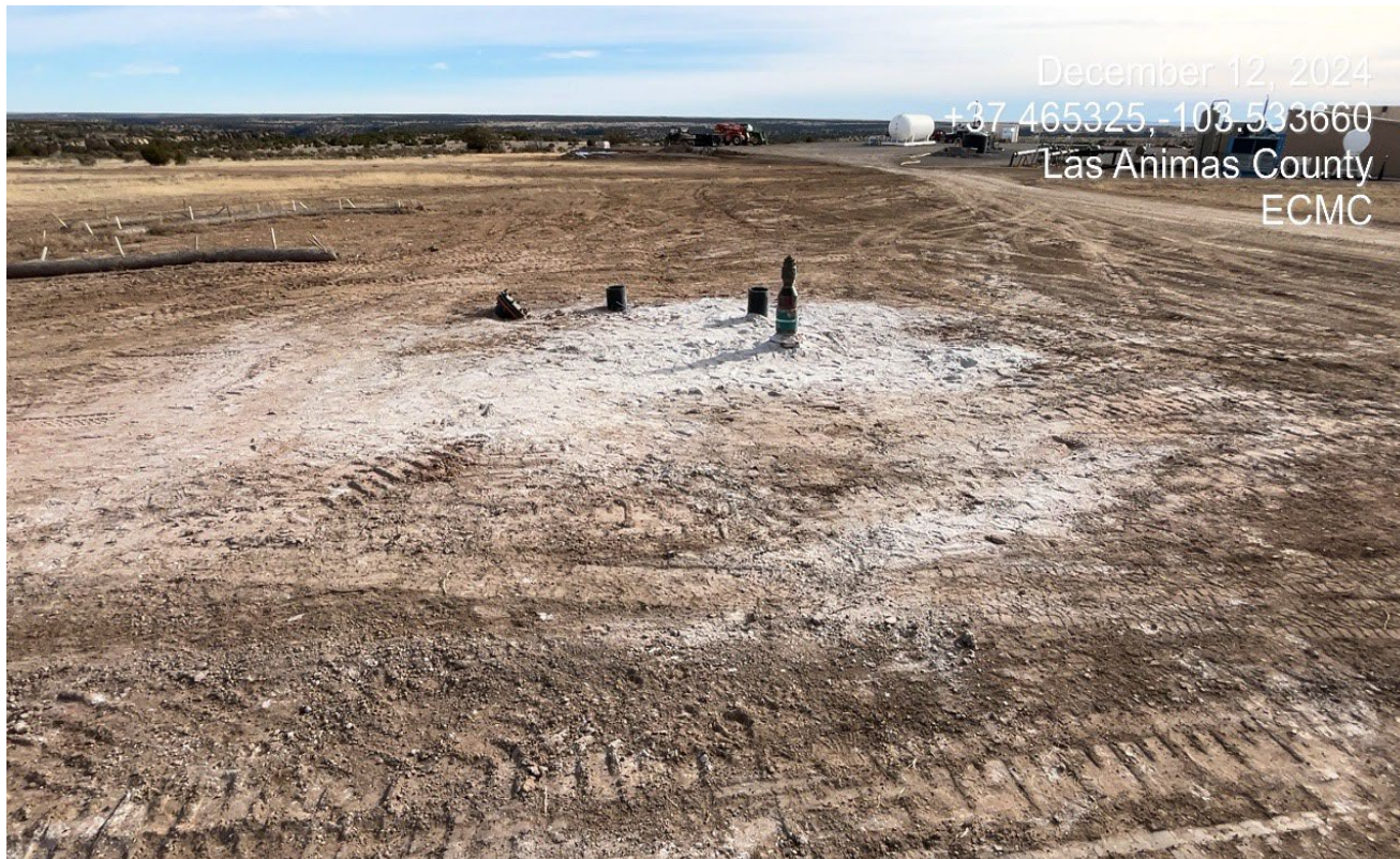
Photo 4. Facing toward the wellsite. There is white material waste around the well that must be cleaned up and properly disposed..
