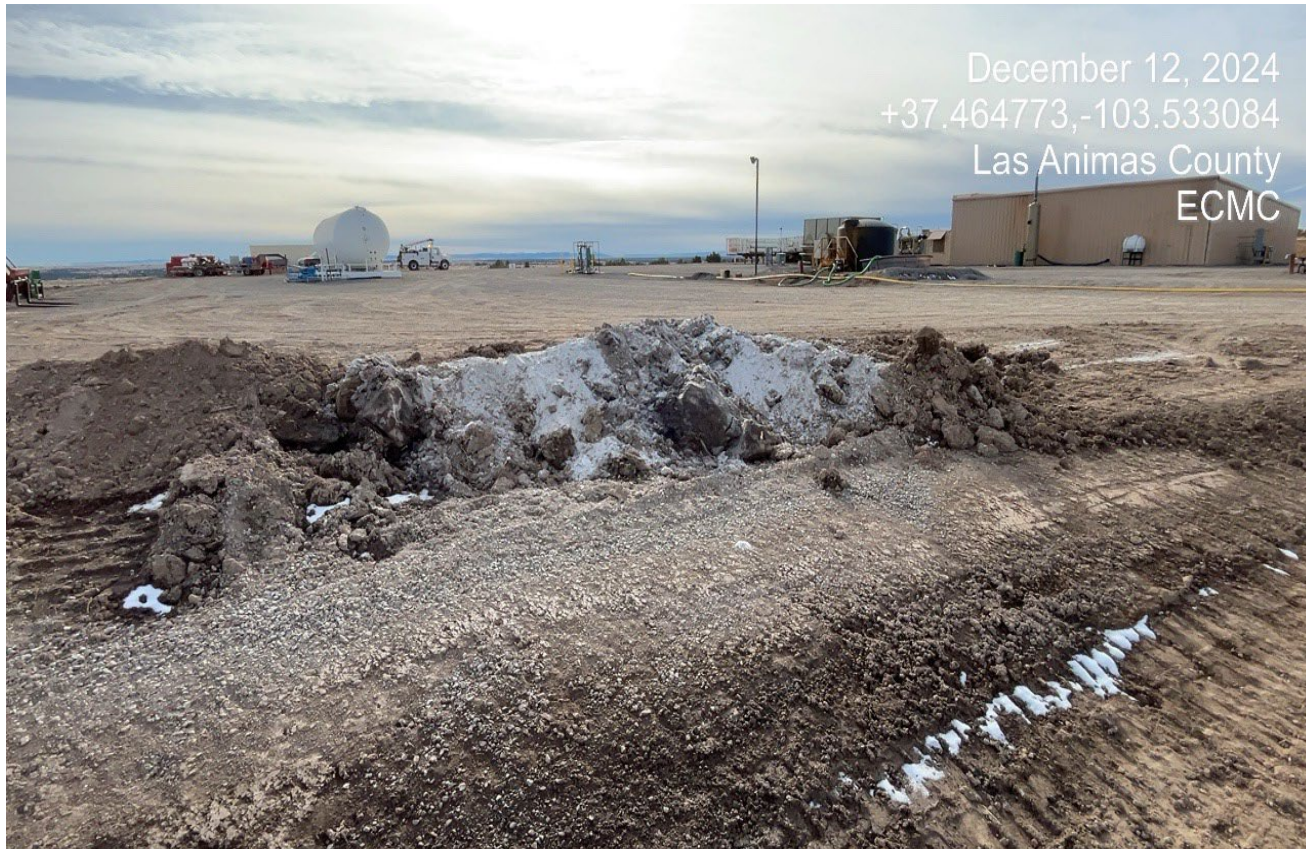
Photo 8. Facing toward the gas plant. There is a whit material that pushed and mixed in with soil which is adjacent to the wellsite. All waste material needs to be cleaned up and properly disposed.
