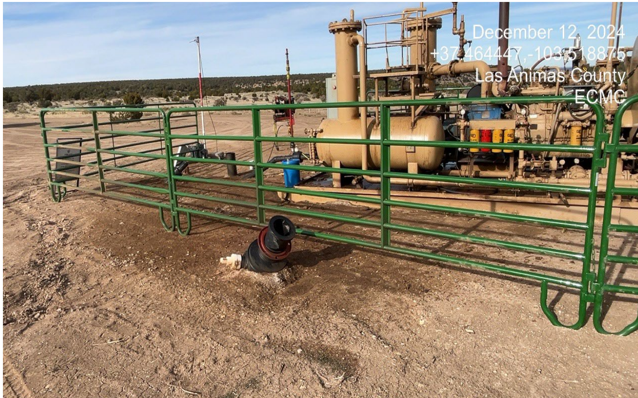
Photo 4. Facing northwest at the wellsite. Stained oily soils sprayed out on both side of the compressor.
