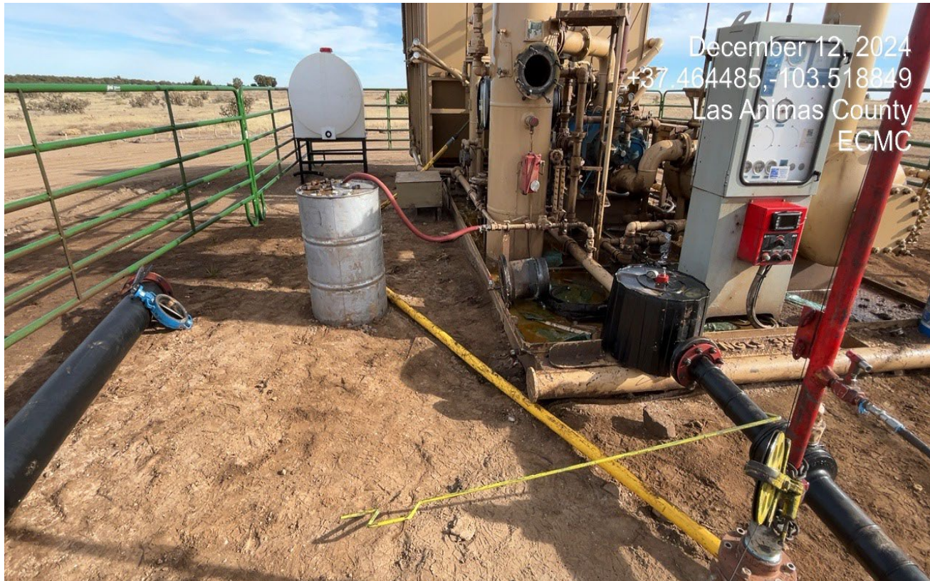
Photo 6. There is oil fluid inside the engine skid that must be cleaned up. The grey drum needs to be placed into secondary containment and labeled.
