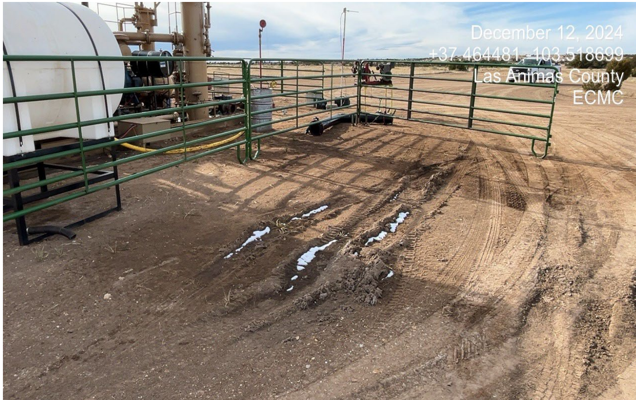
Photo 5. North side of the compressor facing west. Stained oily soils sprayed out on both side of the compressor. Vehicles are driving thru and tracking this area.
