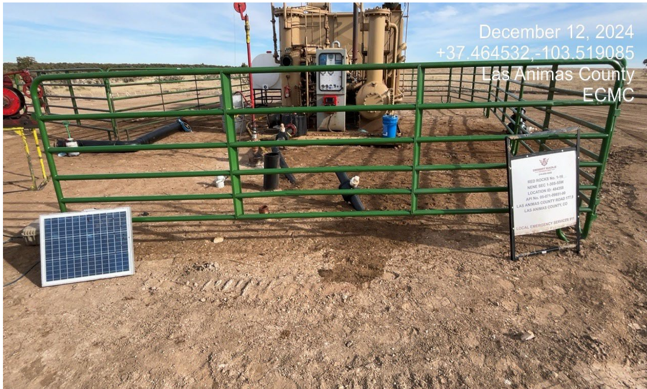
Photo 3. There is dark stained soils at the wellsite and engine compressor. Impacted soils need immediate clean up.
