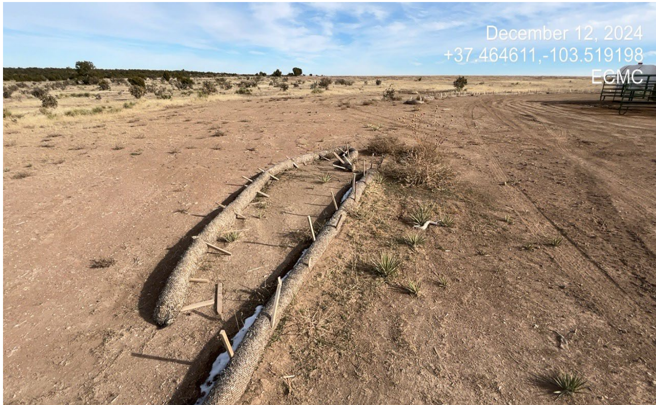
Photo 8. North side of the location facing east/ The wattles have been displaced and need to be reinstalled.
