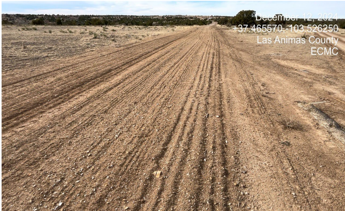
Photo 2. Facing back west toward the flowline disturbance. The vegetation is not establishing along the flowline. It appears this area was reseeded however, soils need to be stabilized with BMP's such as mulch ect.
