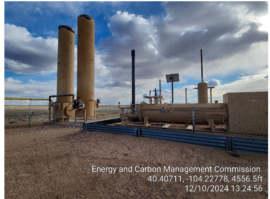
Photo 6 – ECDs and Separator
