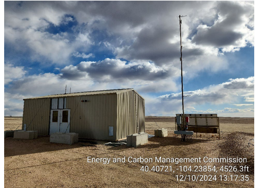
Photo 4 – Gas Lift Injection Meter House
