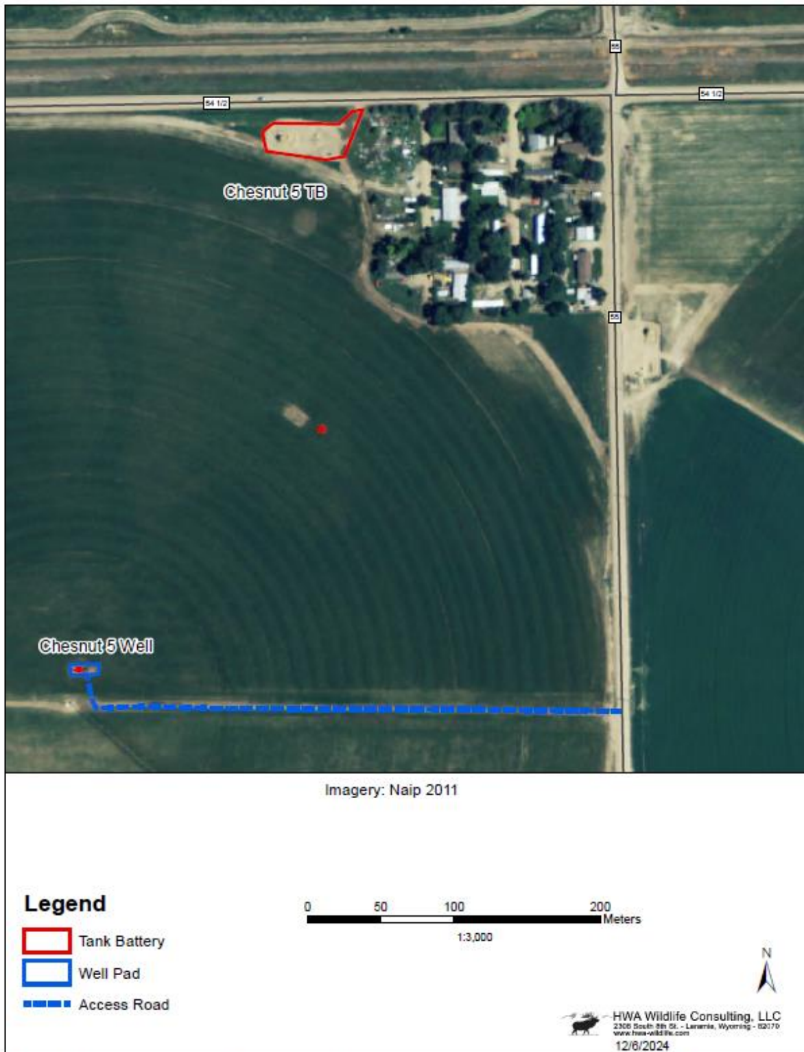
Figure 2. Pre-plugging overview of the reclaimed well site and the associated access road, tank battery, and flowline.
