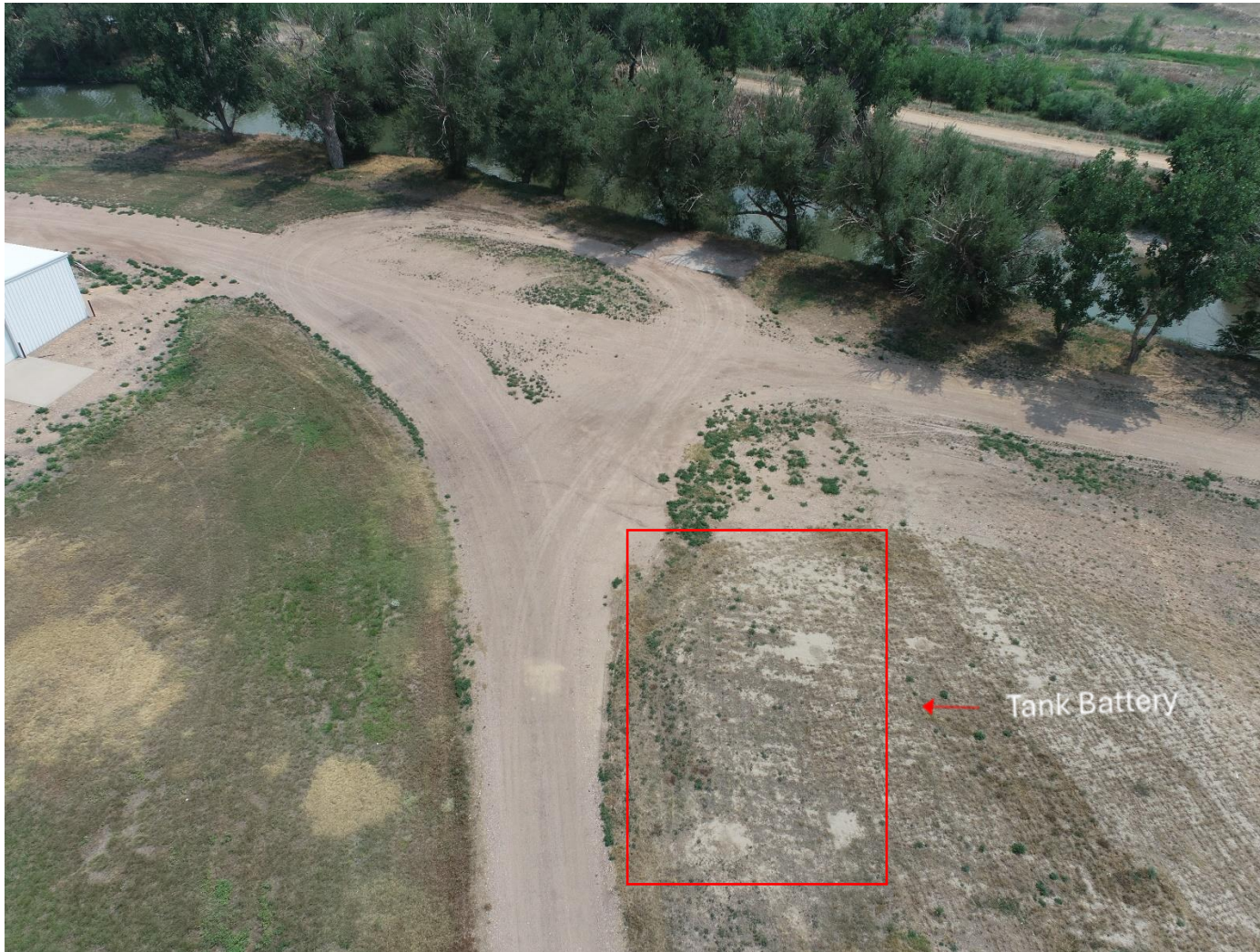
Figure 11: Looking South towards TB, 100 feet in height, Lat/Long: 40.422009/-104.646799. Ground Photos (7/22/2024):
