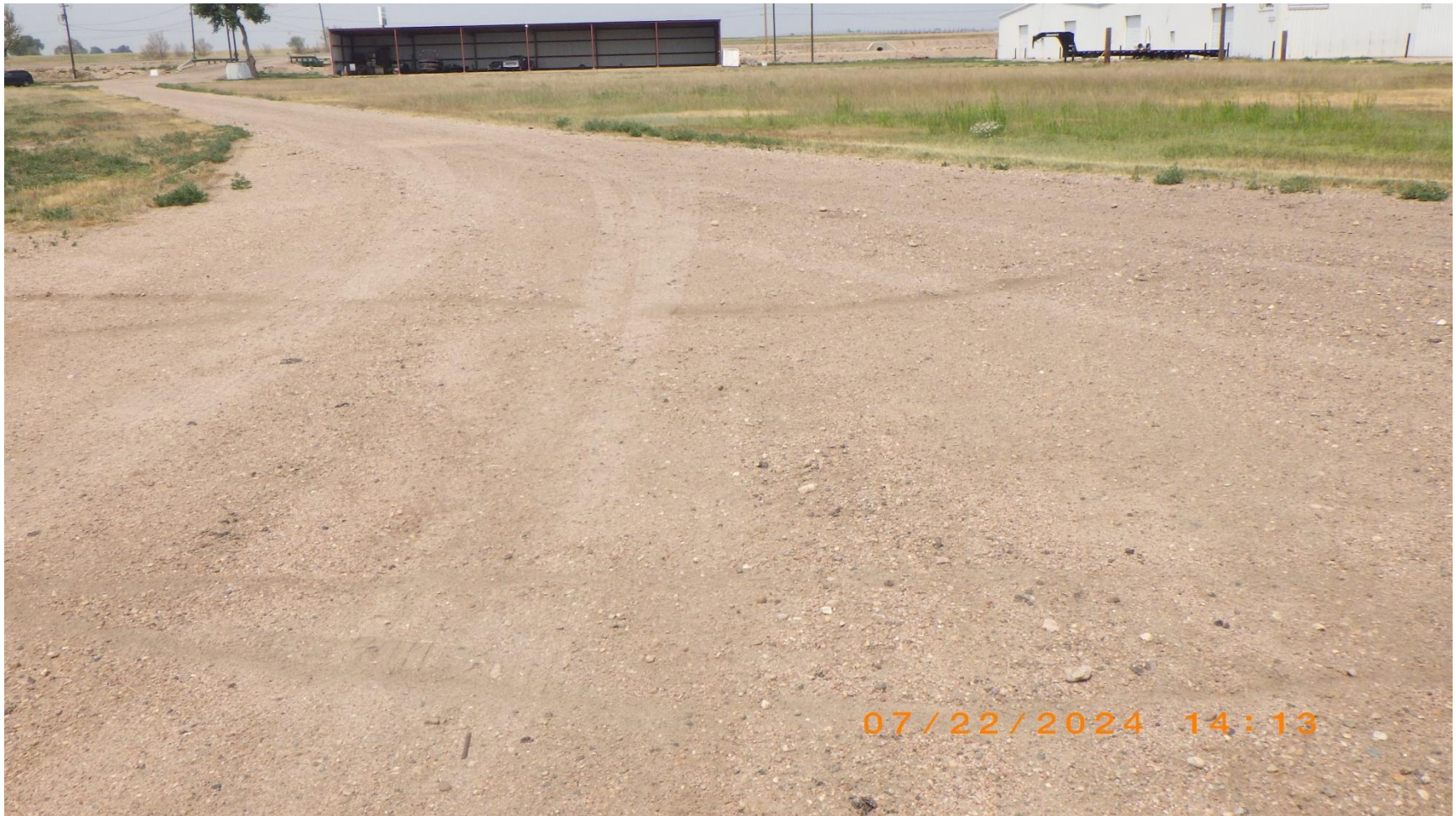
Figure 18: South edge of TB looking North.
