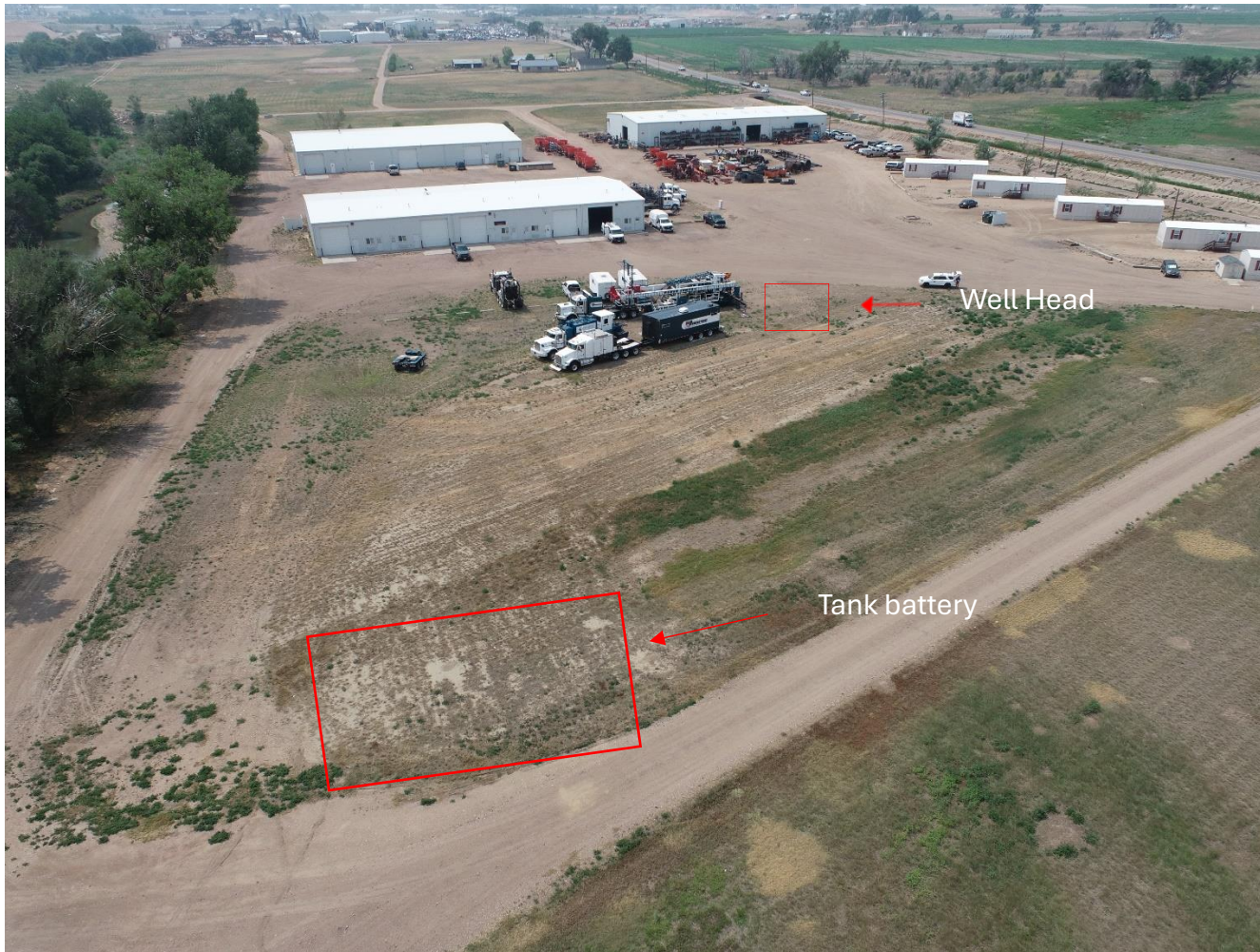
Figure 6: Looking West towards well and flowline, 100 feet in height, Lat/Long: 40.421652/-104.646307.
