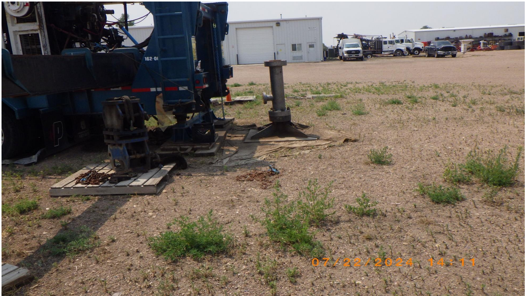
Figure 13: East edge of well looking West.
