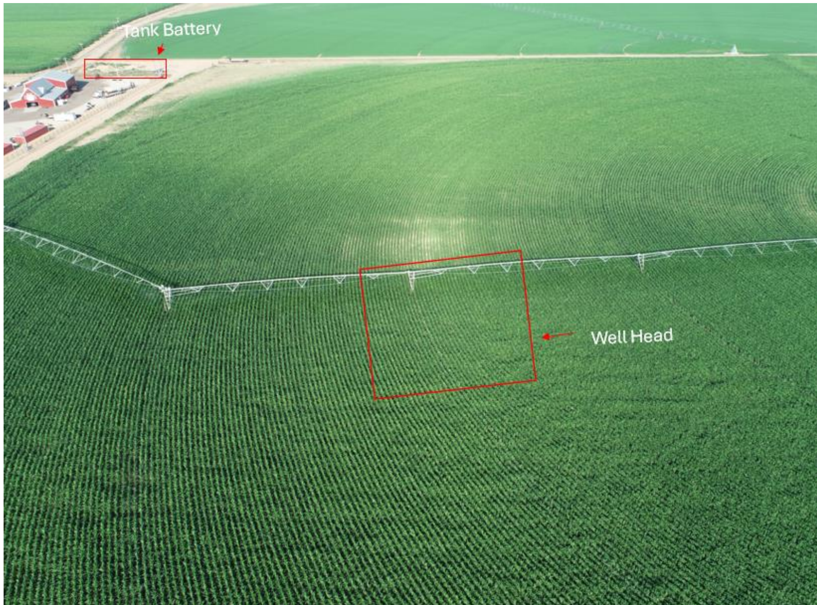
Figure 9: Looking West towards the Flowline, 200 feet in height, Lat/Long: 40.532589/-104.659815.
