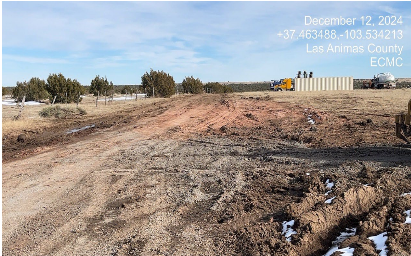
Photo 9. Standing on County Road 179 facing east toward DEO property. There is red drill cutting sand that has been spread on the road at Lat/Long:37.40116,-103.51736. E&P waste from the wellsite was not properly disposed.
