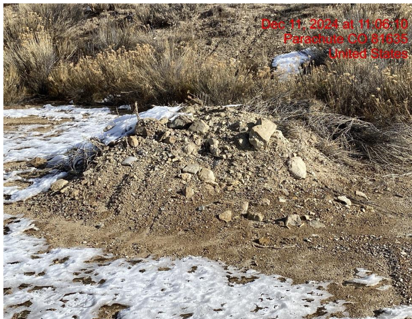
Unprotected Soil Stockpile – Photo #05255
