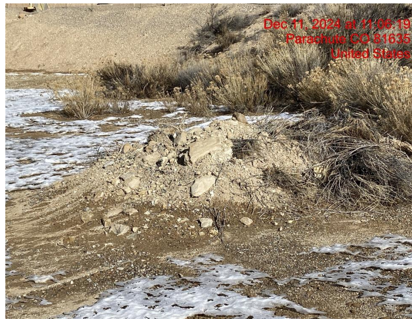
Unprotected Soil Stockpile – Photo #05256
