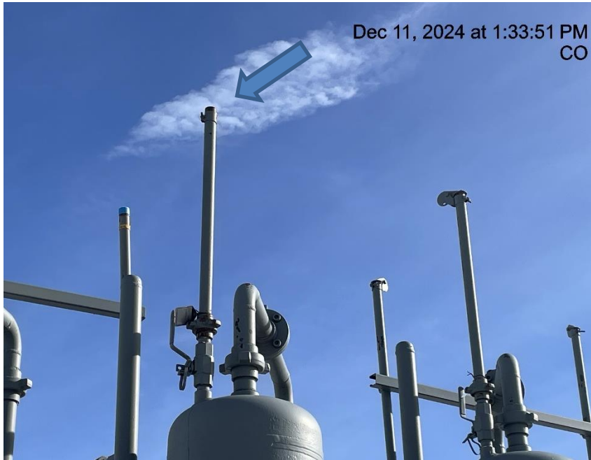
Photo # 3176 Rupture disc vent line does not comply with CECMC pressure safety device rules
