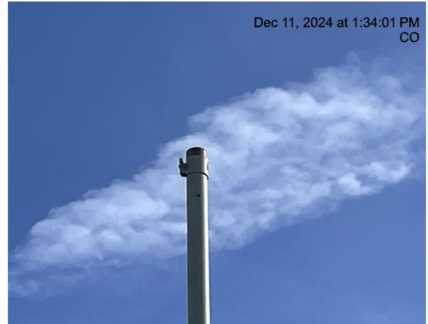
Photo # 3177 Rupture disc vent line does not comply with CECMC pressure safety device rules
