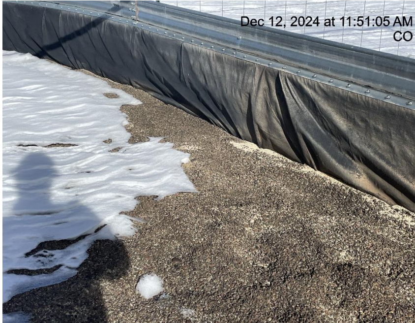
Photo # 3479 Staining in secondary containment
