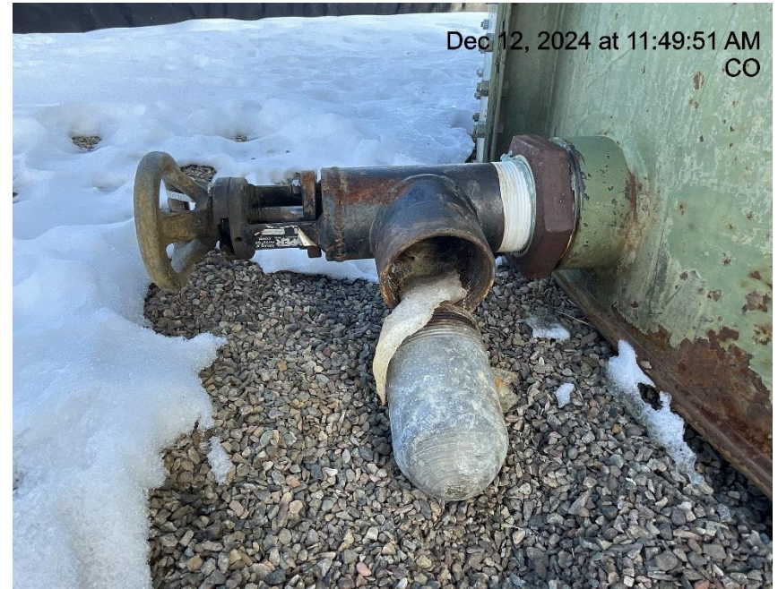
Photo # 3478 Open ended load line
