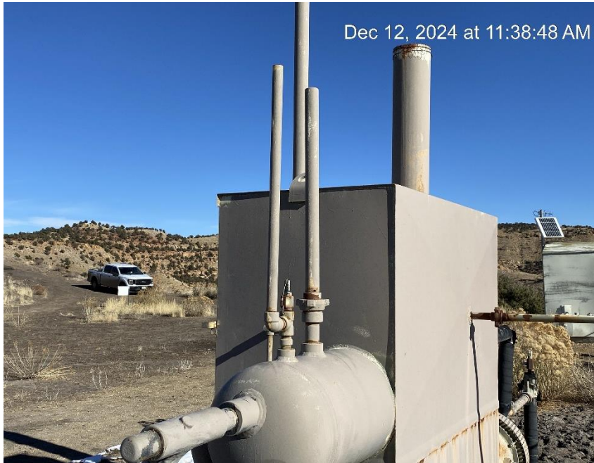
Caps missing on relief vent risers
