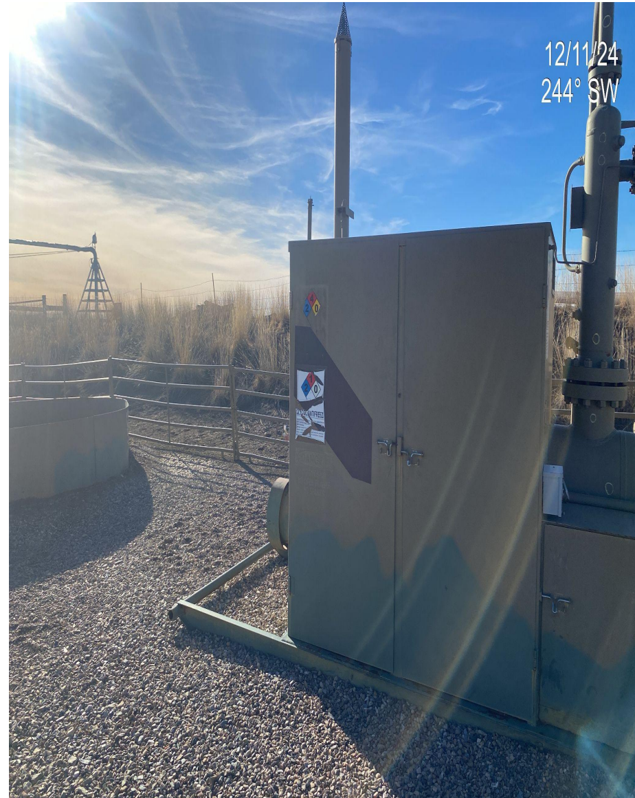
Photo 2. Placards/Signs at separators are deteriorating, future maintenance is advised.
