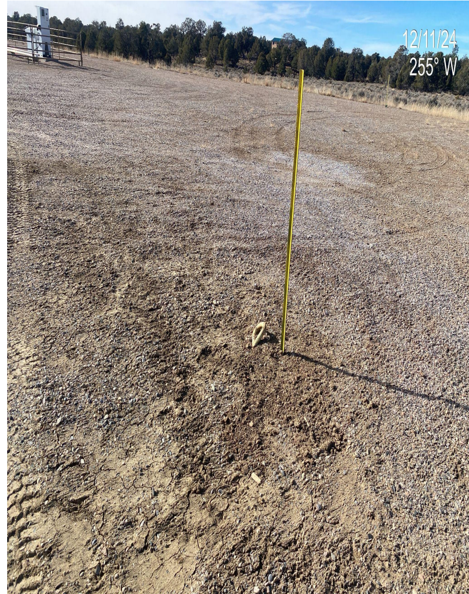
Photo 4. Marked guyline anchors on the active pad.
