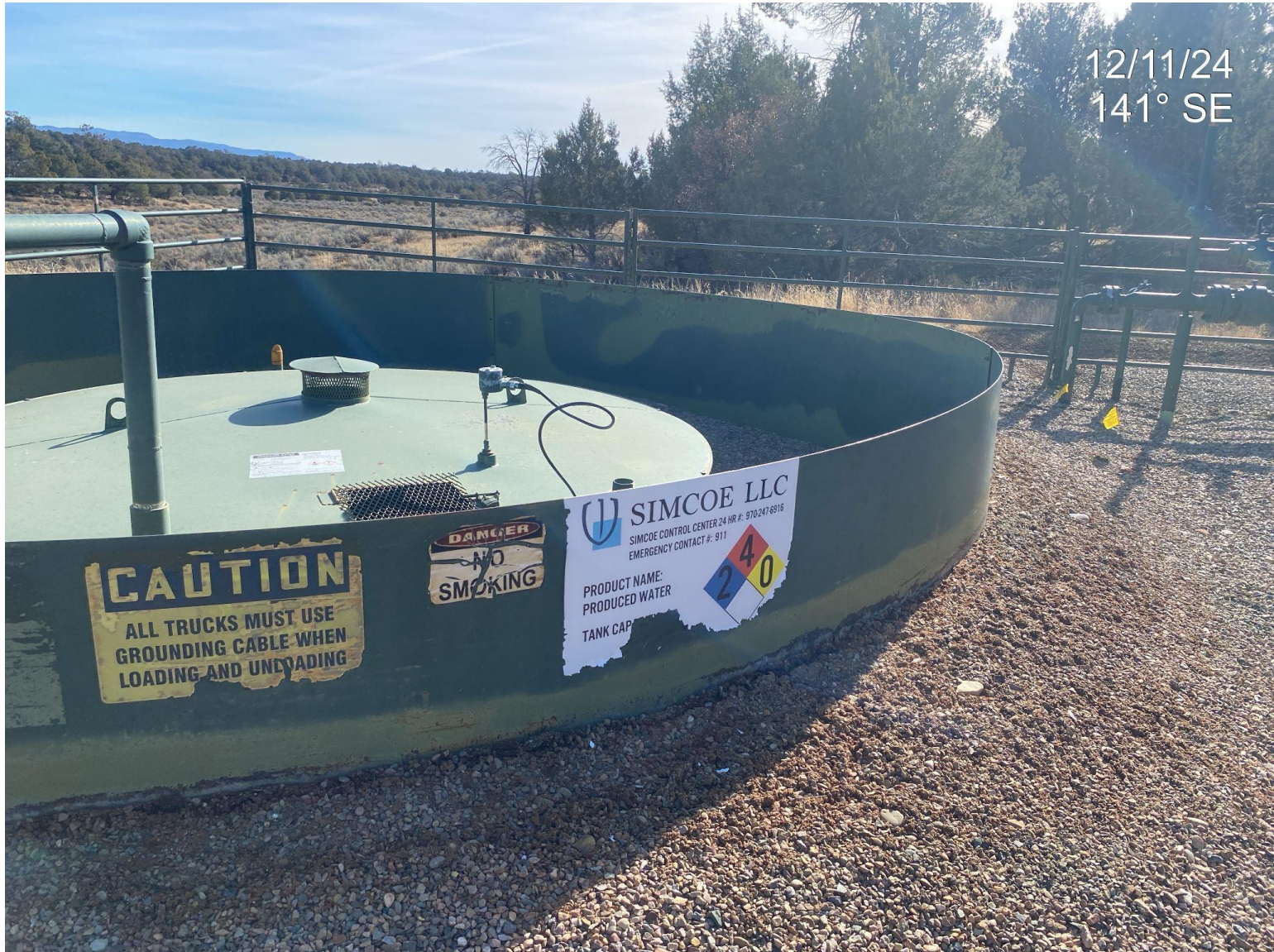
Photo 3. Produced water tank label/placard deteriorating and no longer displaying capacity.
