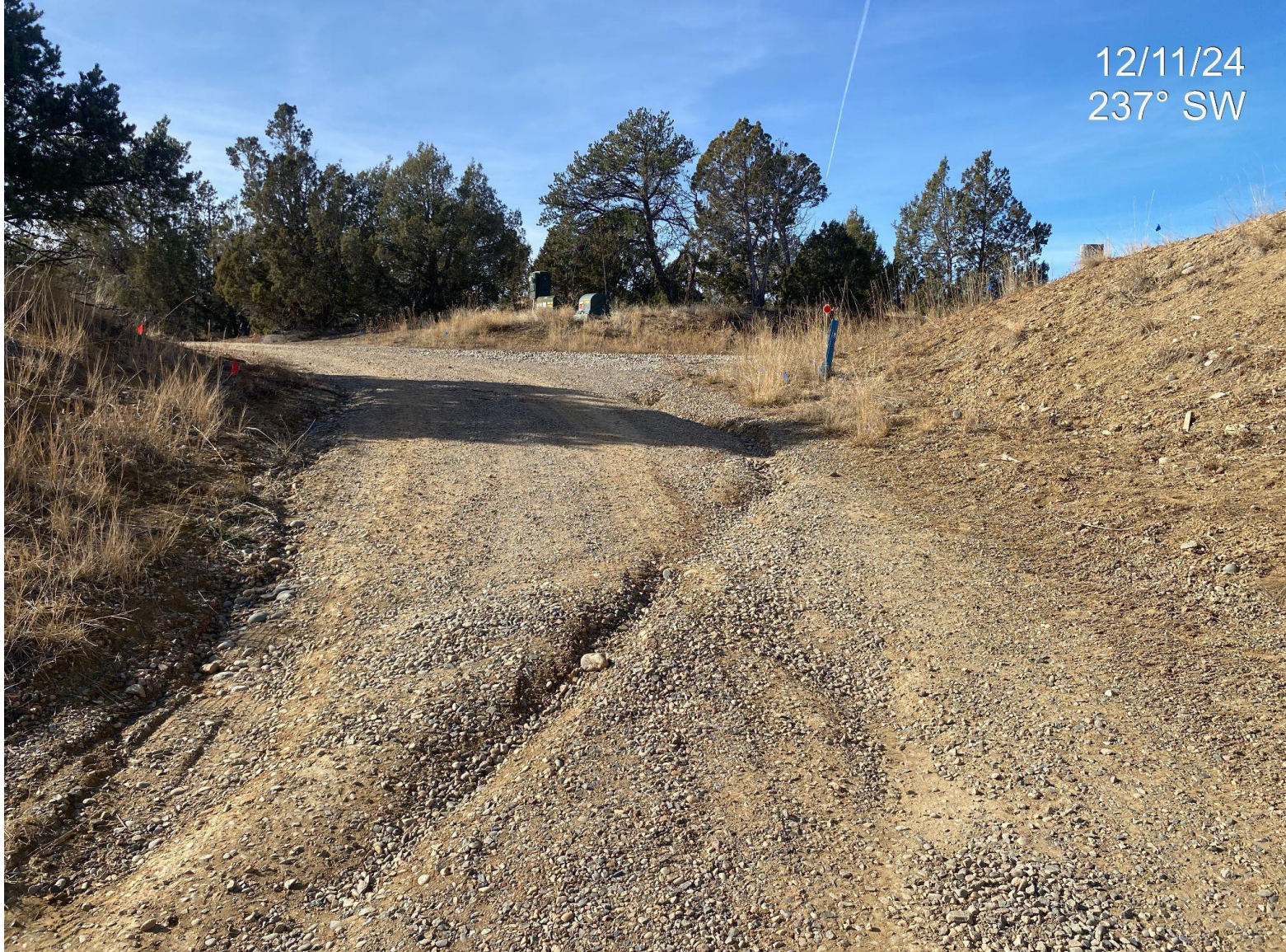
Photo 3. Erosion starting to form at the access point, future maintenance is advised.
