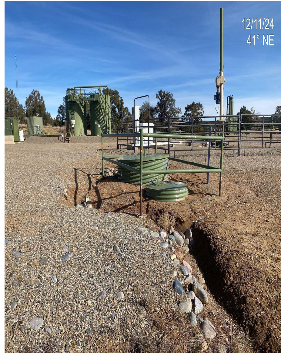
Photo 4. Gully erosion forming on the southern edge of the active pad.
