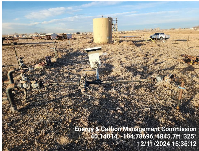
Photo 9 Gas Meter Run.
