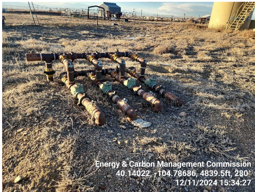
Photo 7 Flow line manifold.
