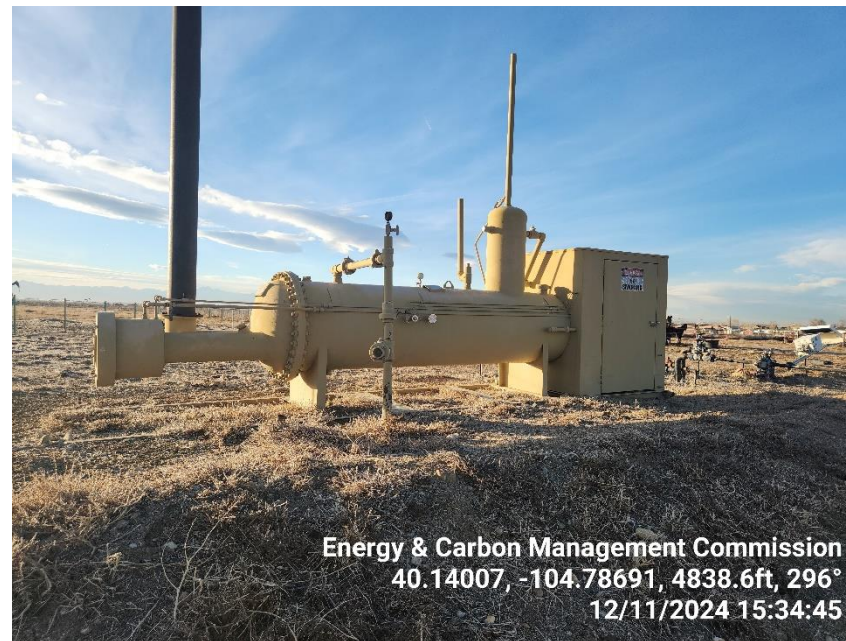
Photo 8 Horizontal Heated Separator.
