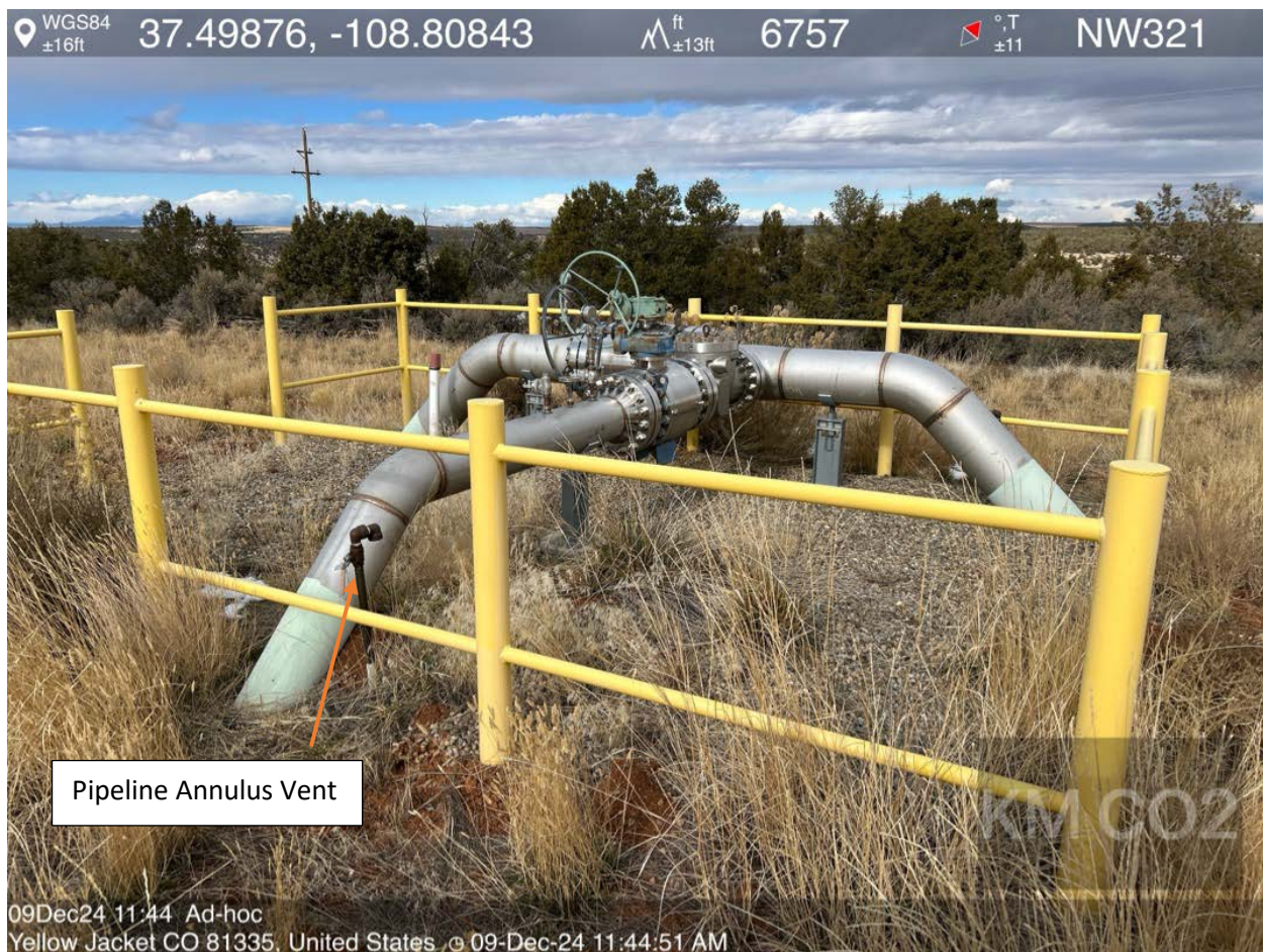
Photo #6. View of above-ground YE-YF Loop Manifold which is located due north of the existing bollard cage (Photos #1 & #2). The pipeline annulus vent visible in the foreground of this photo has a tag that is labeled "YE Loop" and "Annulus Vent"
