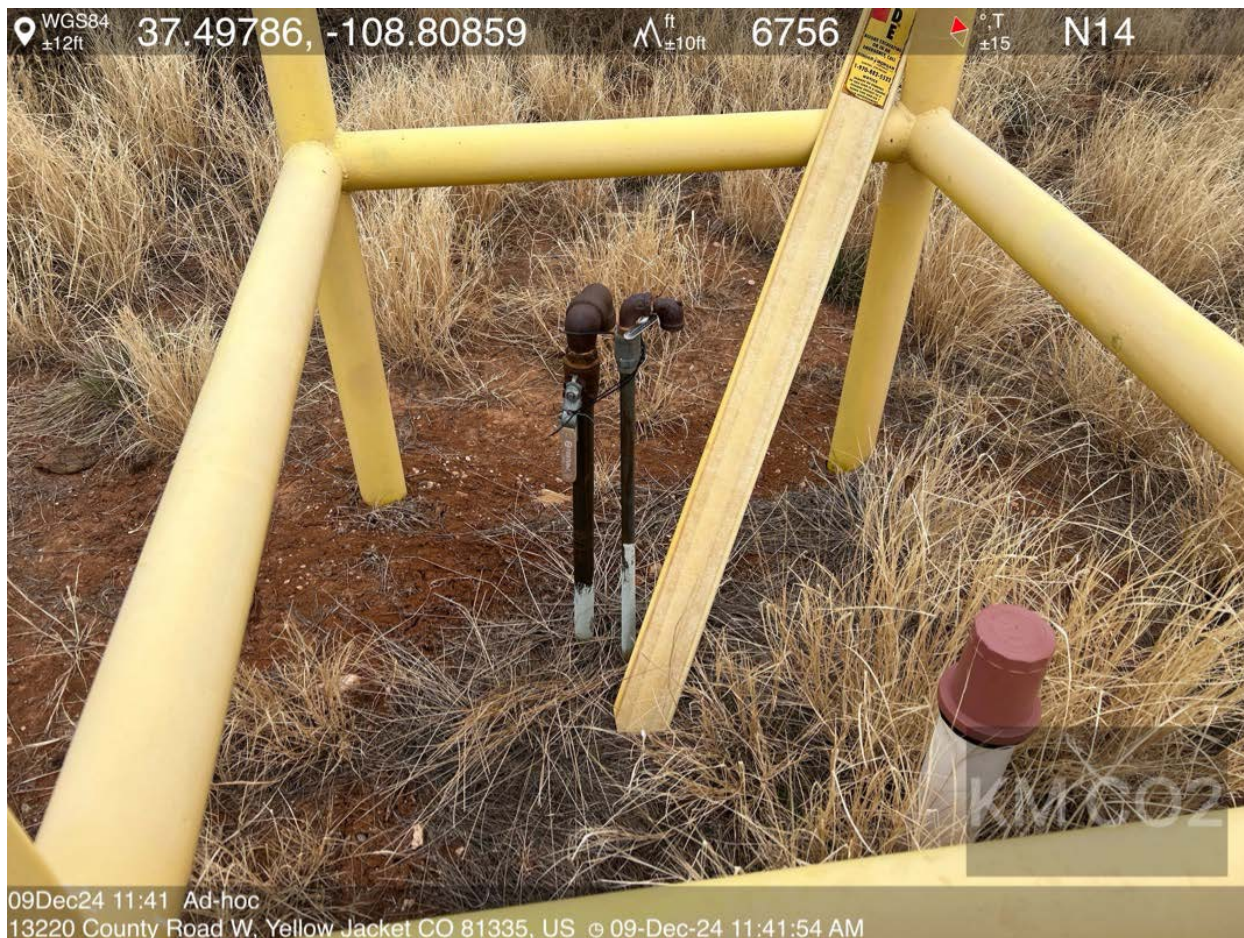
Photo #2. Close up view of the pipeline annulus vents supporting the YE Loopline near the YE-7 P&A well location.
