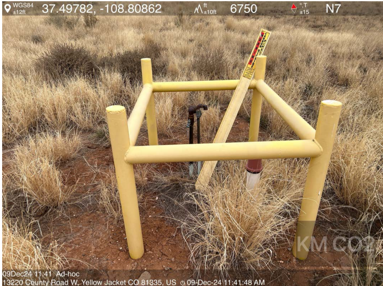
Photo #1. View of above ground bollard cage, pipeline annulus vents, and corrosion protection sleeve located adjacent to the YE-7 P&A well location.
