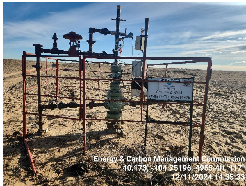
Photo 2 Wellhead & sign.
