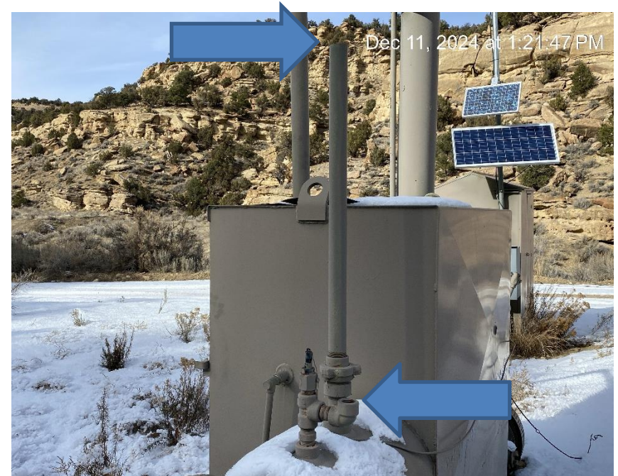
Relief vent riser caps missing
