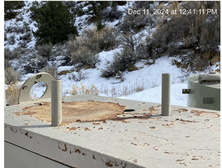
Relief vent riser caps missing
