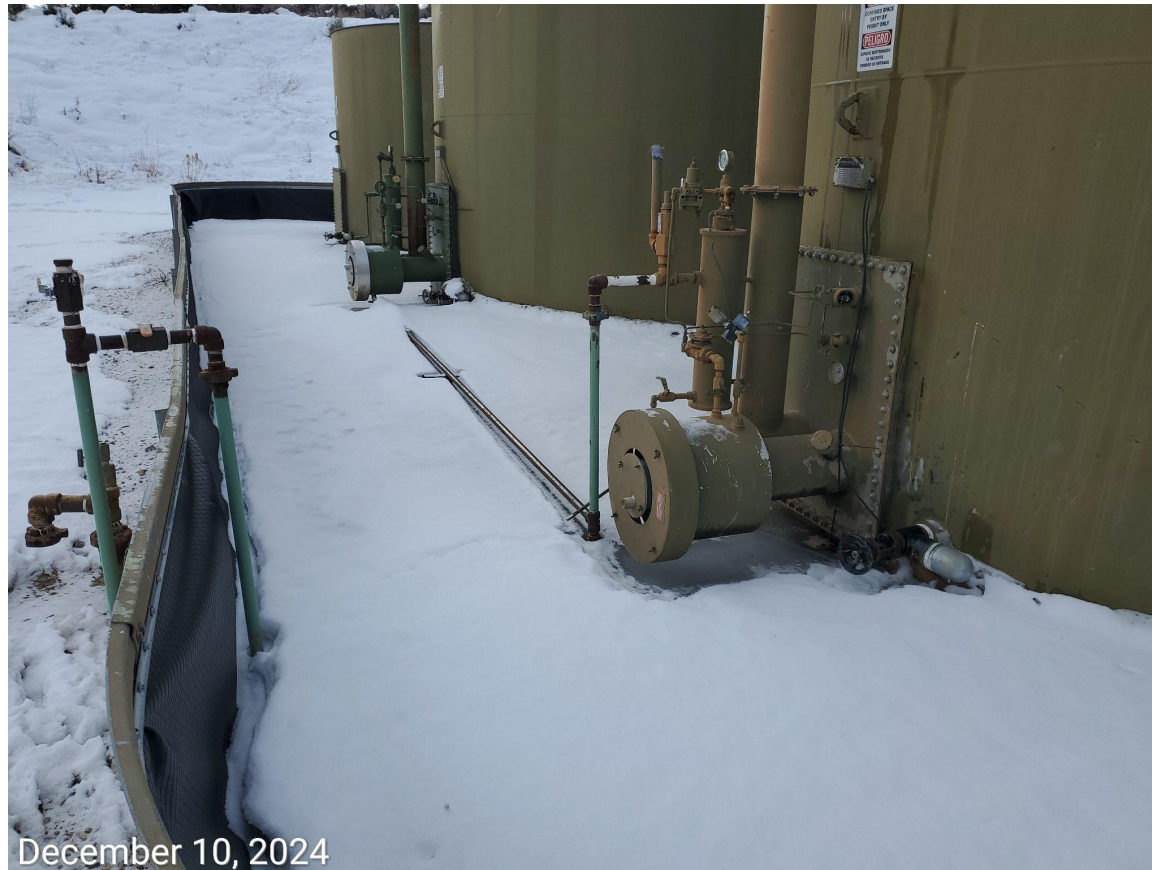
Photo 2: Lines at tanks have been capped/plugged.
