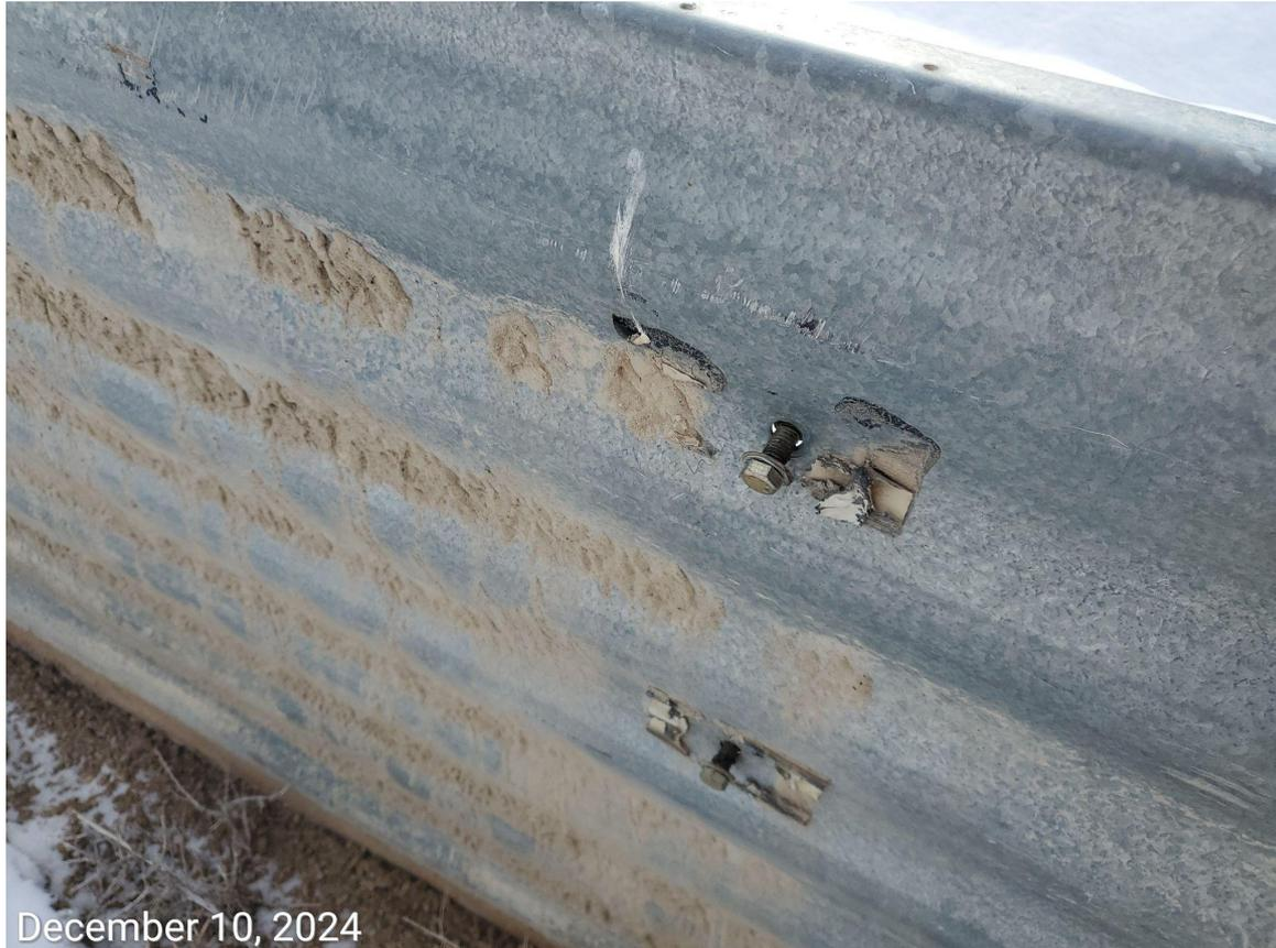
**Photo 5:** Photo taken from the secondary containment measure at the battery. Photo shows Operator has loosely placed bolts within the holes observed in the metal walls; BMP remains inadequate to contain a spill or release.
