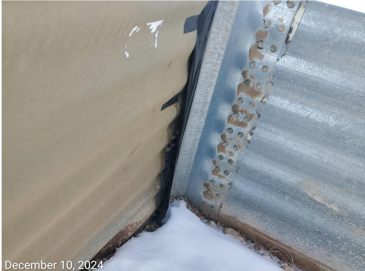
**Photo 2:** Photo taken from the secondary containment measure at the battery. Photo shows Operator appears to have placed electrical tape within compromised areas of at the containment BMP; tape is peeling from the metal; BMP remains inadequate to contain a spill or release.
