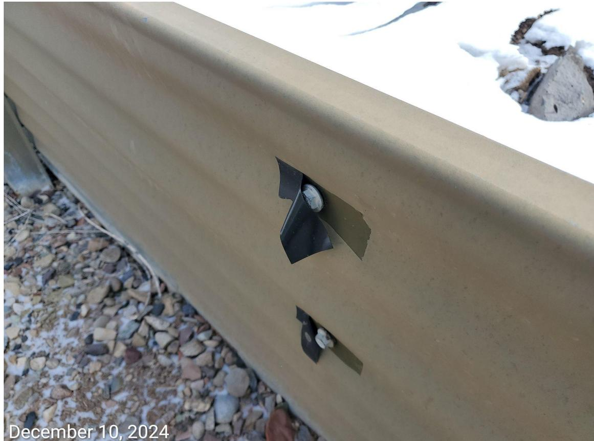
**Photo 7:** Photo taken from the secondary containment measure at the battery. Photo shows Operator has placed loose bolts within holes, and what appears electrical tape within compromised areas of at the containment BMP; BMP remains inadequate to contain a spill or release.
