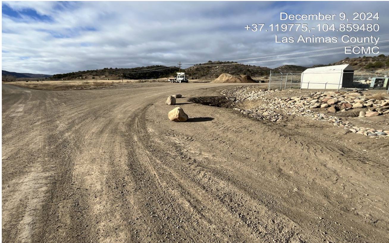
Photo 1. Facing southwest along the main road to the A.C. Tank Battery. A sediment ahs been installed along the road side. The rock barriers may be obscured during snow accumulation. Reflector markers may be more suited at this area.
