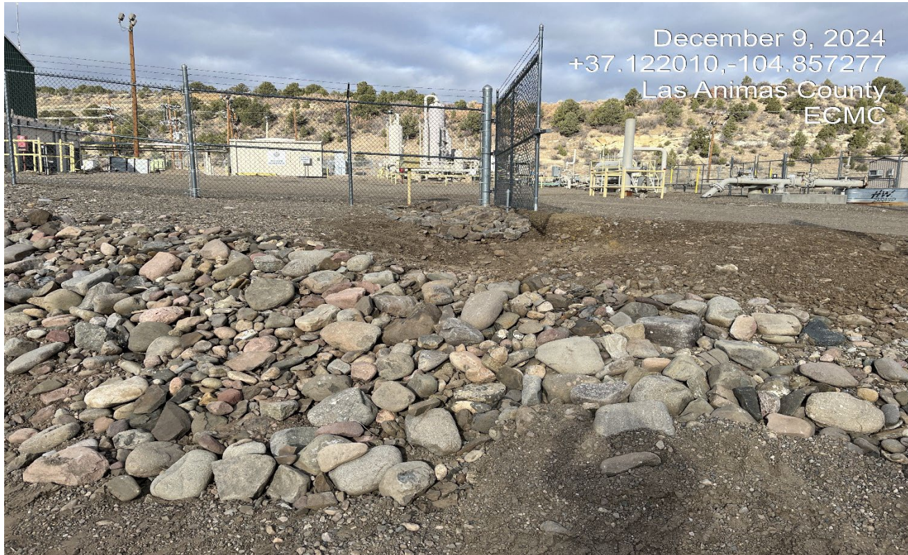
Photo 2. A sediment trap was installed to prevent erosion onto the road.
