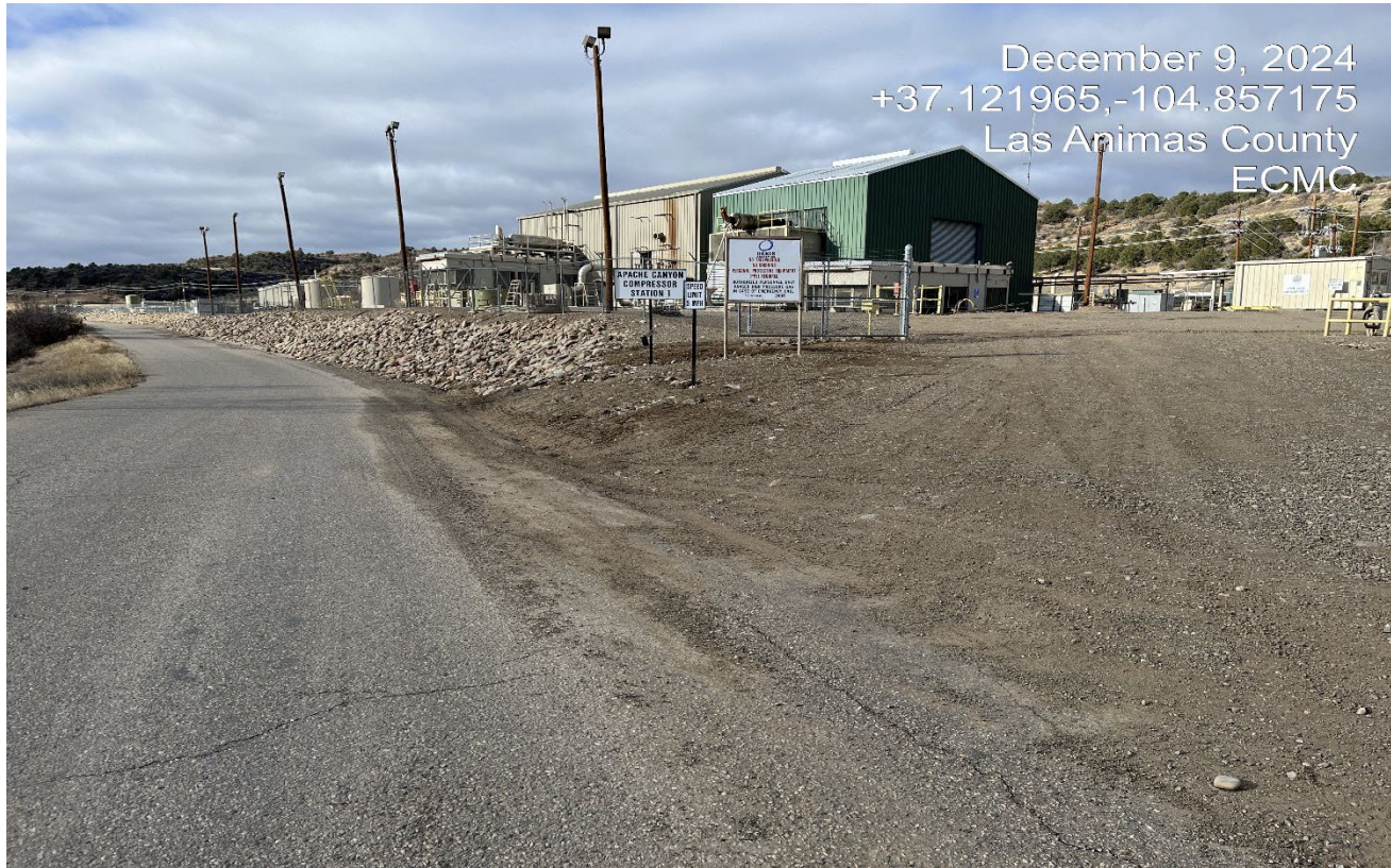
Photo 1. Facing southwest along the main road to the compressor facility.
