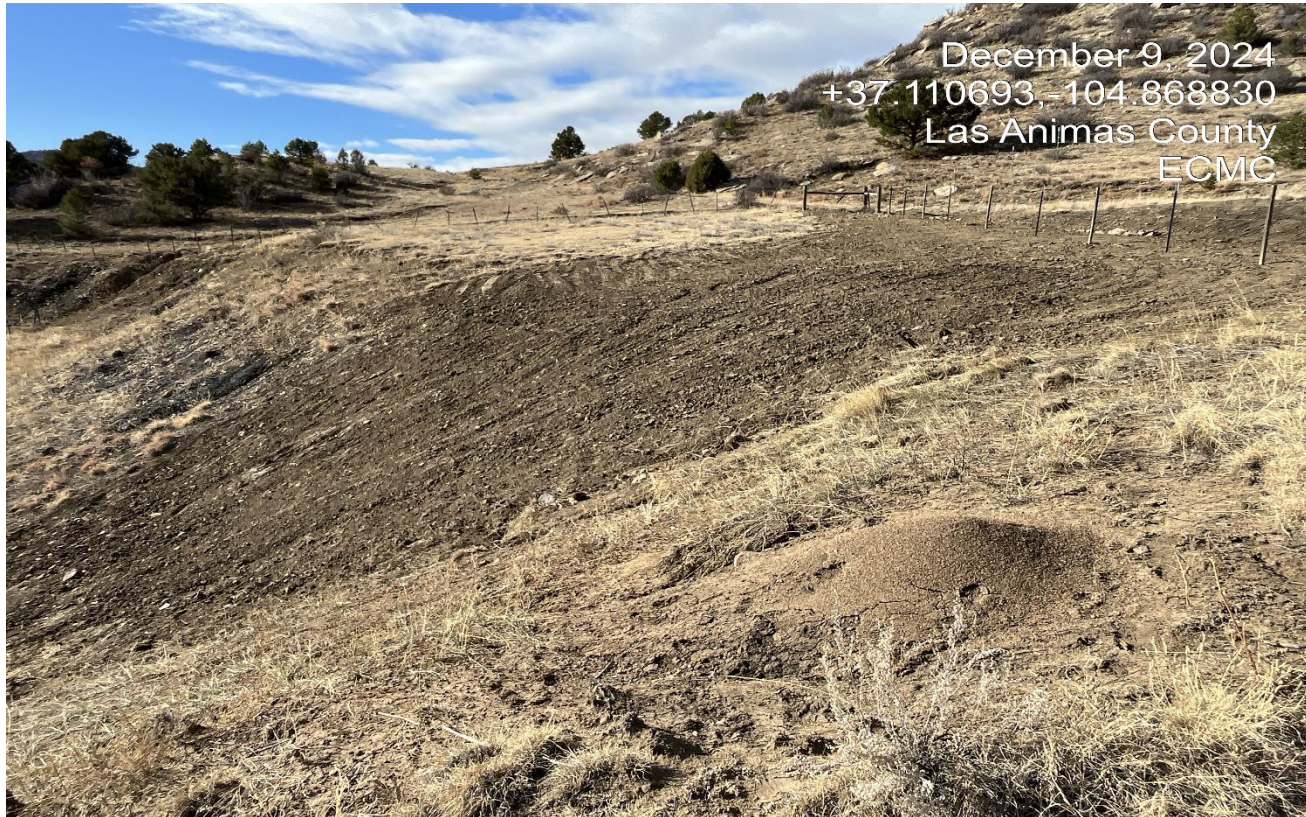
Photo 3. The erosion gully along the cut slope has been repaired.
