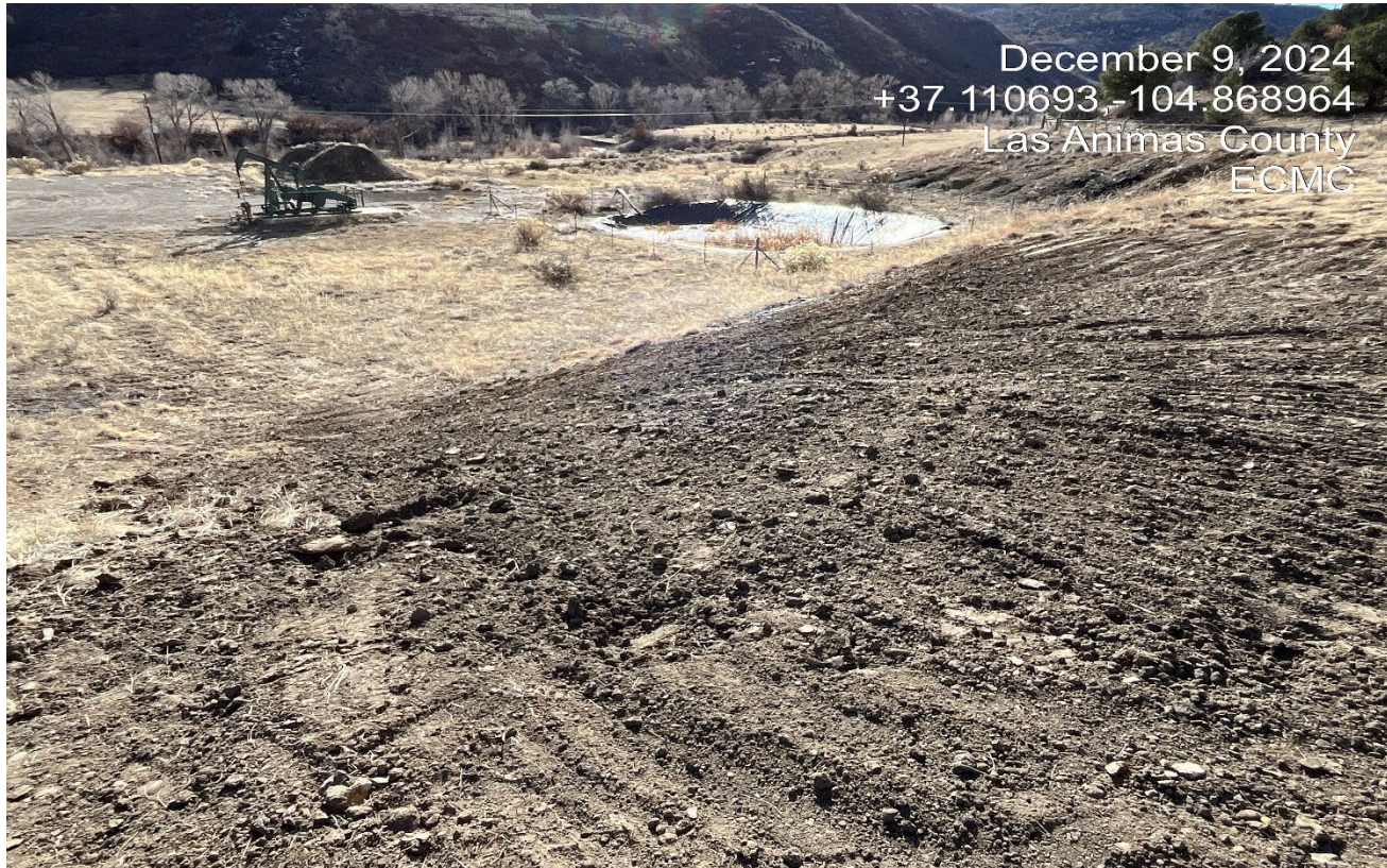
Photo 5. Facing toward the erosion repair. It appears the excavator teeth were dragged downhill along the slope which will promote erosion. Tracking or grading should be performed perpendicular to the slope to prevent erosion.
