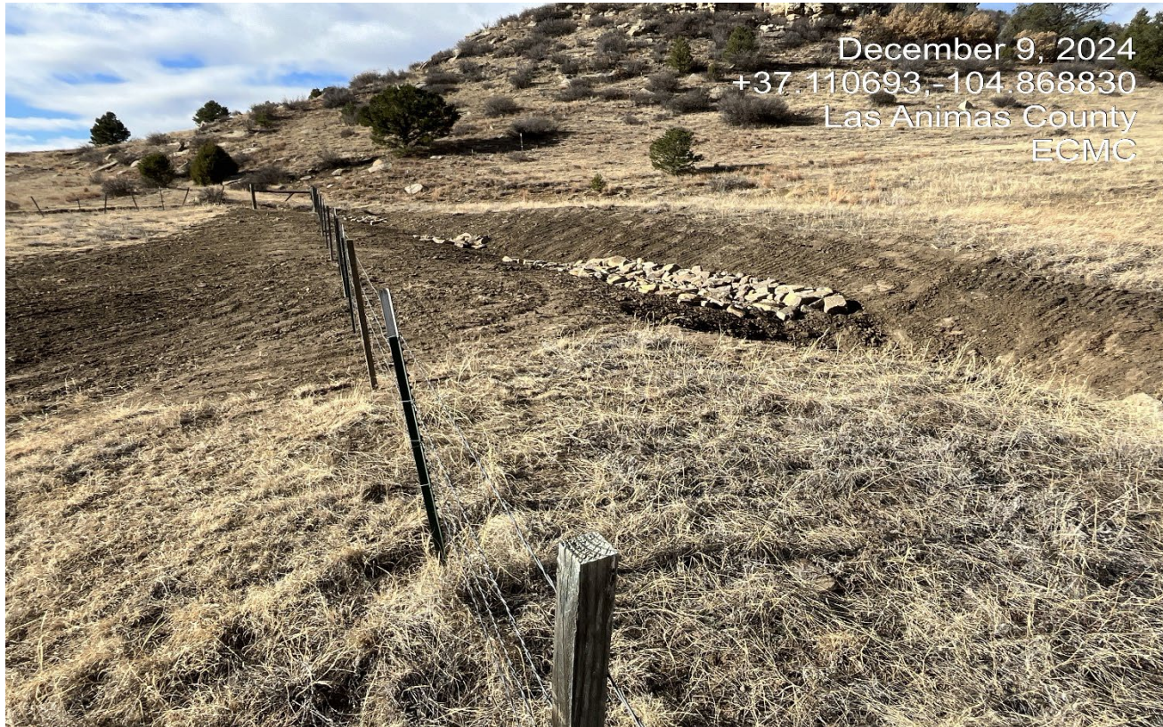
Photo 4. There is a run-of swale above the location that has been graded to promote stormwater away from the cut slope.
