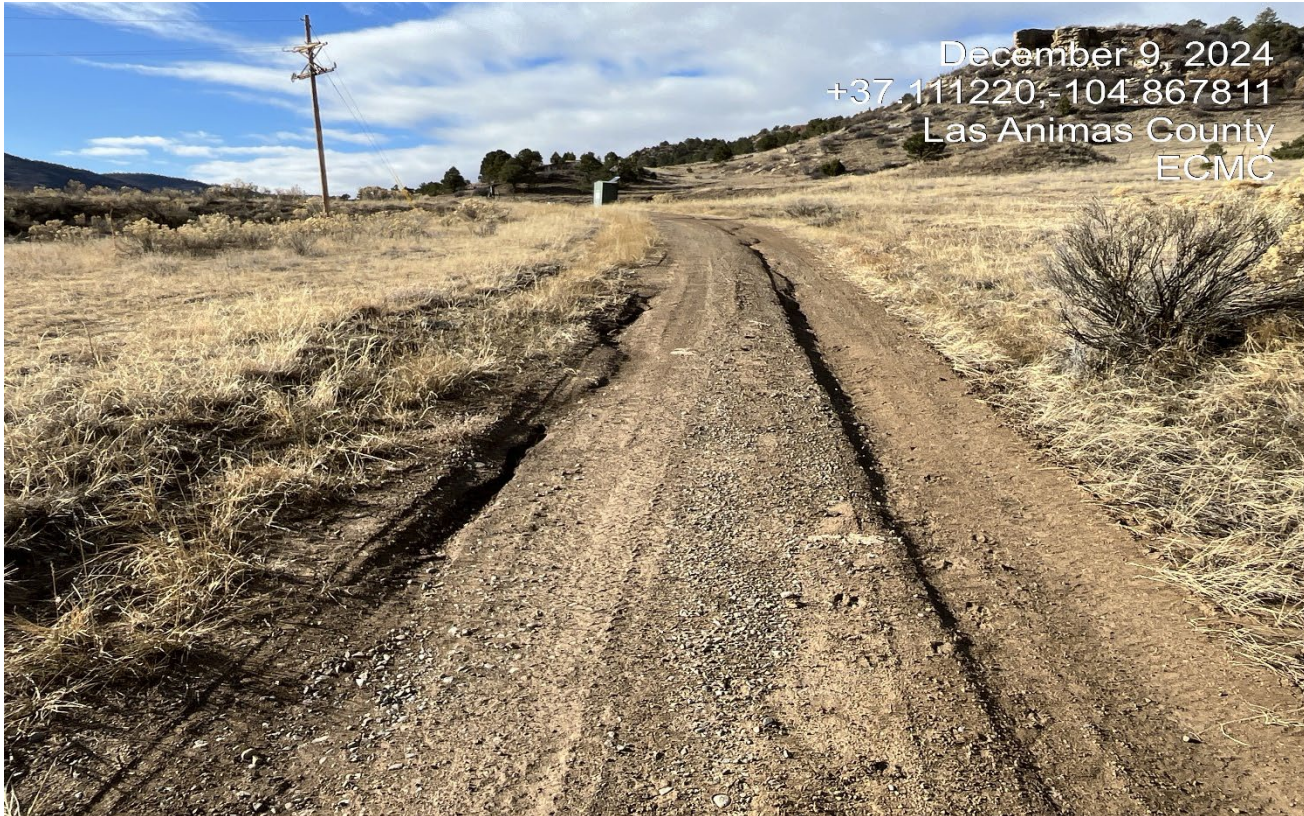
Photo 1. Facing southwest along the access road. There is erosion along the road that needs to be repaired.
