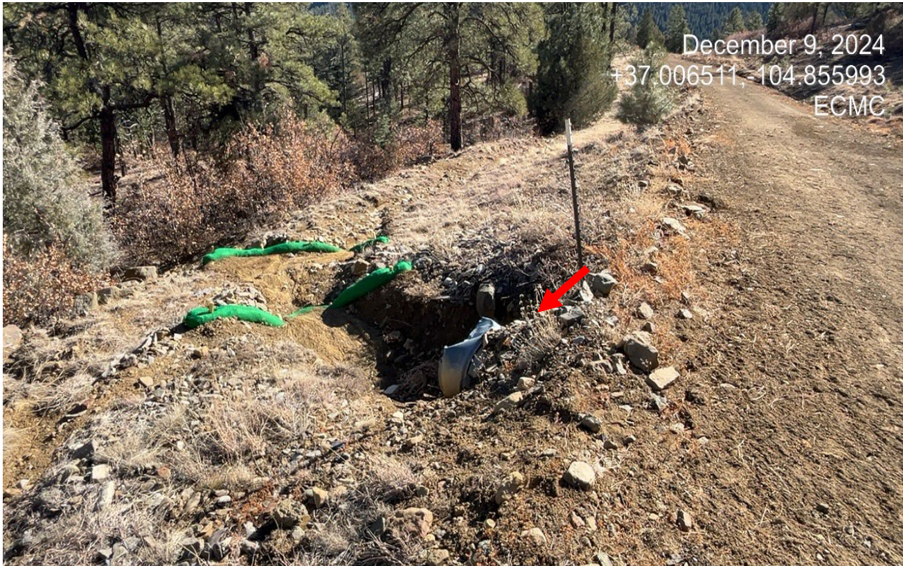
Photo 4. The green wattles were installed at the culvert outlet which has already filled in with sediment. The wattles will need to be cleaned out and sediment control further up the road should be installed.
