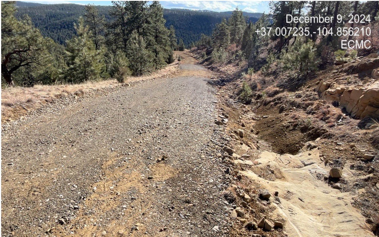
Photo 1. Facing southeast along the access roads. More BMP's need to be installed up along the road to slow down or divert stormwater off the road..
