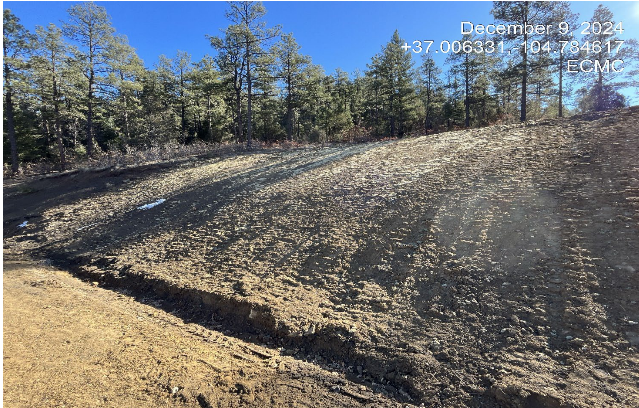
Photo 5. Facing toward the cut slope which has been tracked for temporary stabilization.
