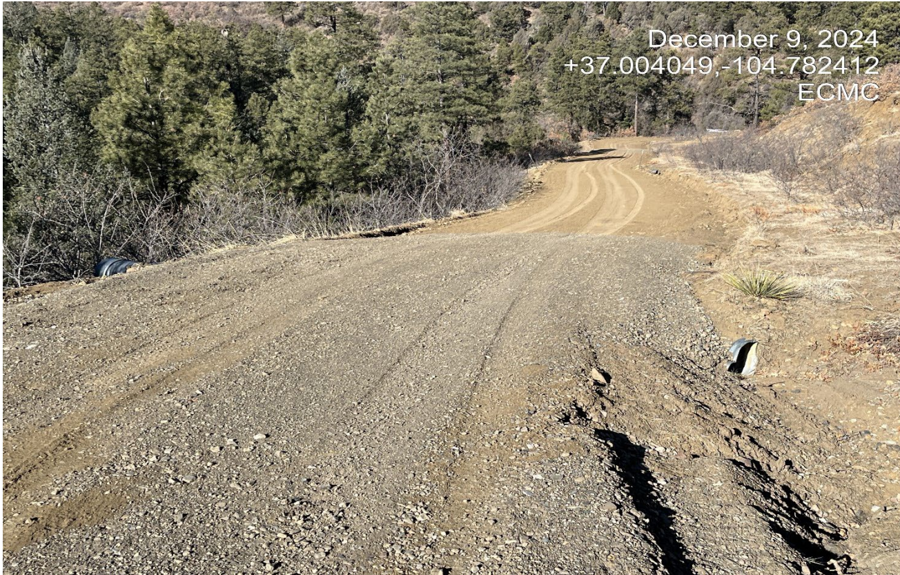
Photo 2. Facing northwest along the road. The culvert has been cleaned out and road base was added to promote drainage off the road.
