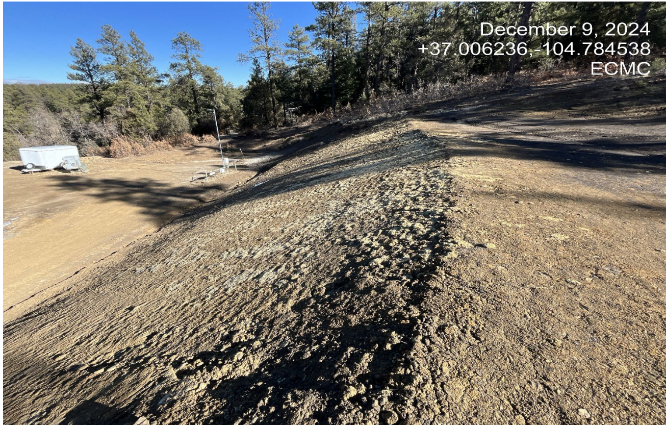
Photo 6. Facing down toward the cut slope. There was some sparse hydromulch spread. It appears work is still in process however hydromulch must be uniformly spread with complete coverage for proper stabilization.
