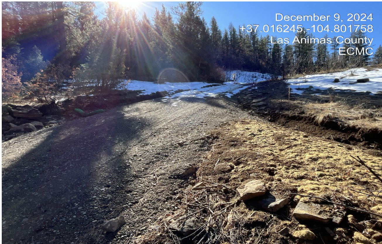
Photo 2. There is a stormwater diversion installed where run-off from the location was occurring. Road base material was hauled into this area for a slight water bar.
