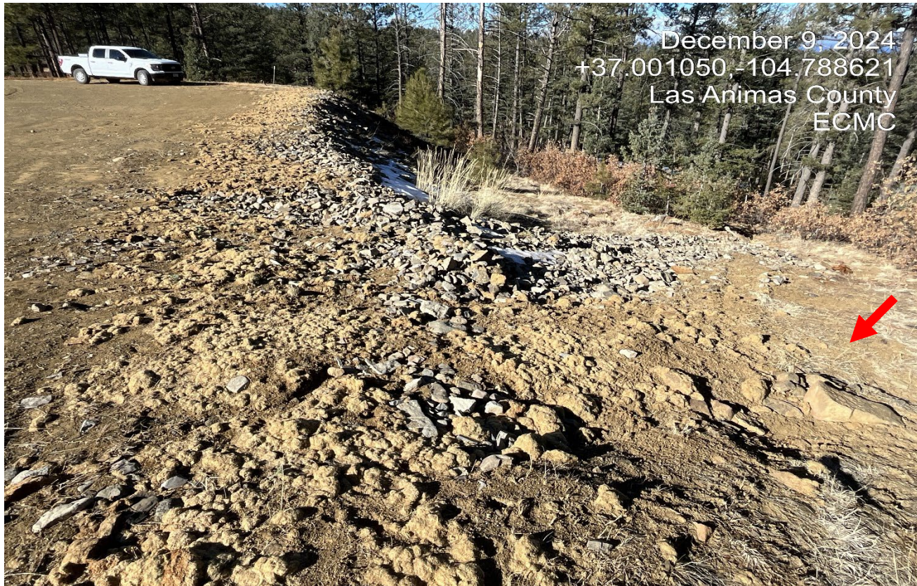
Photo 4. Northeast side of the location facing west. The erosion channels were filled in with rock. Stormwater will find least resistant pathway would could create erosion toward area of red arrow.
