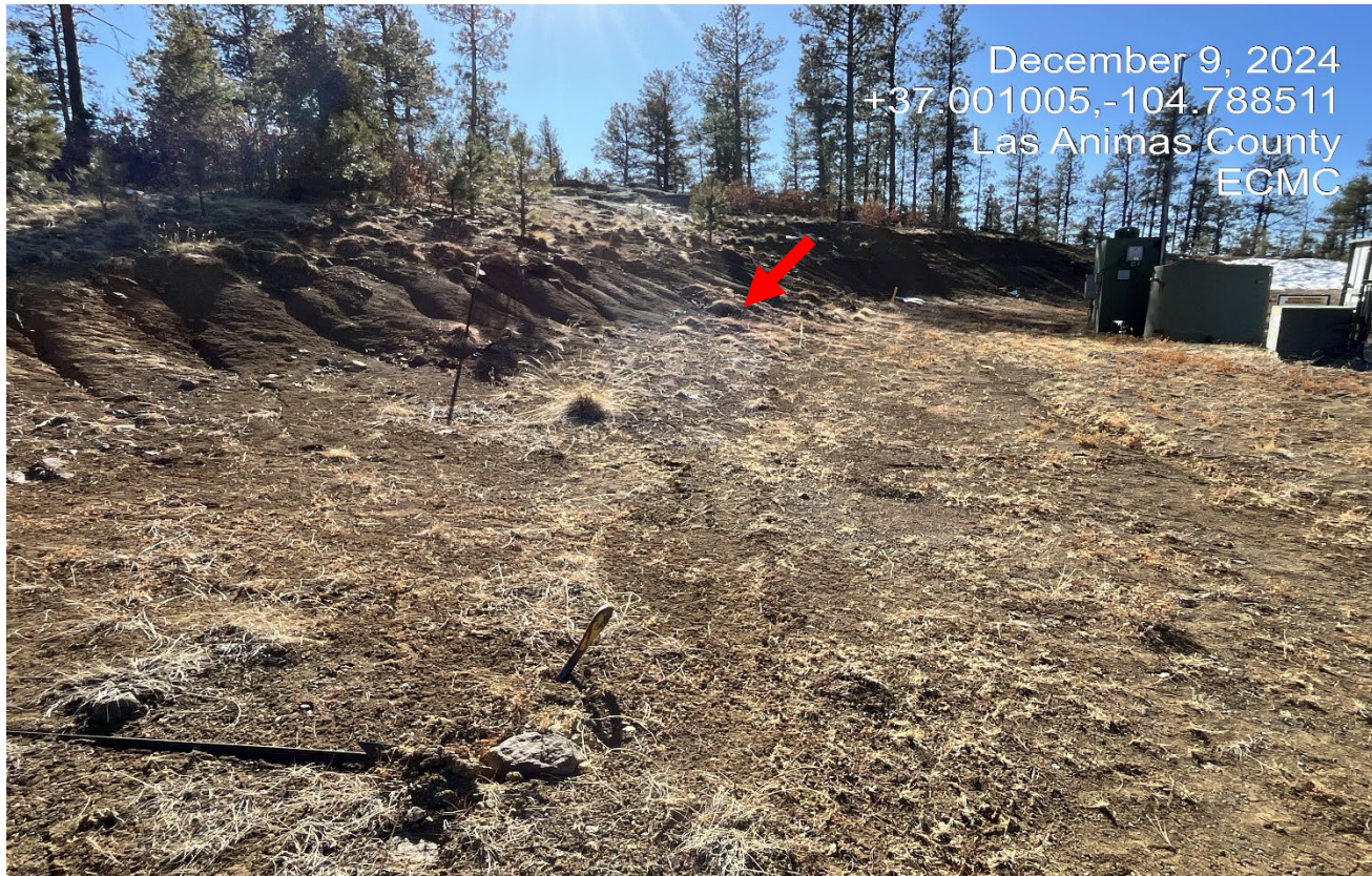
Photo 5. Facing toward the cu slope. There is erosion along the cut slope that needs to be regraded and seeded.
