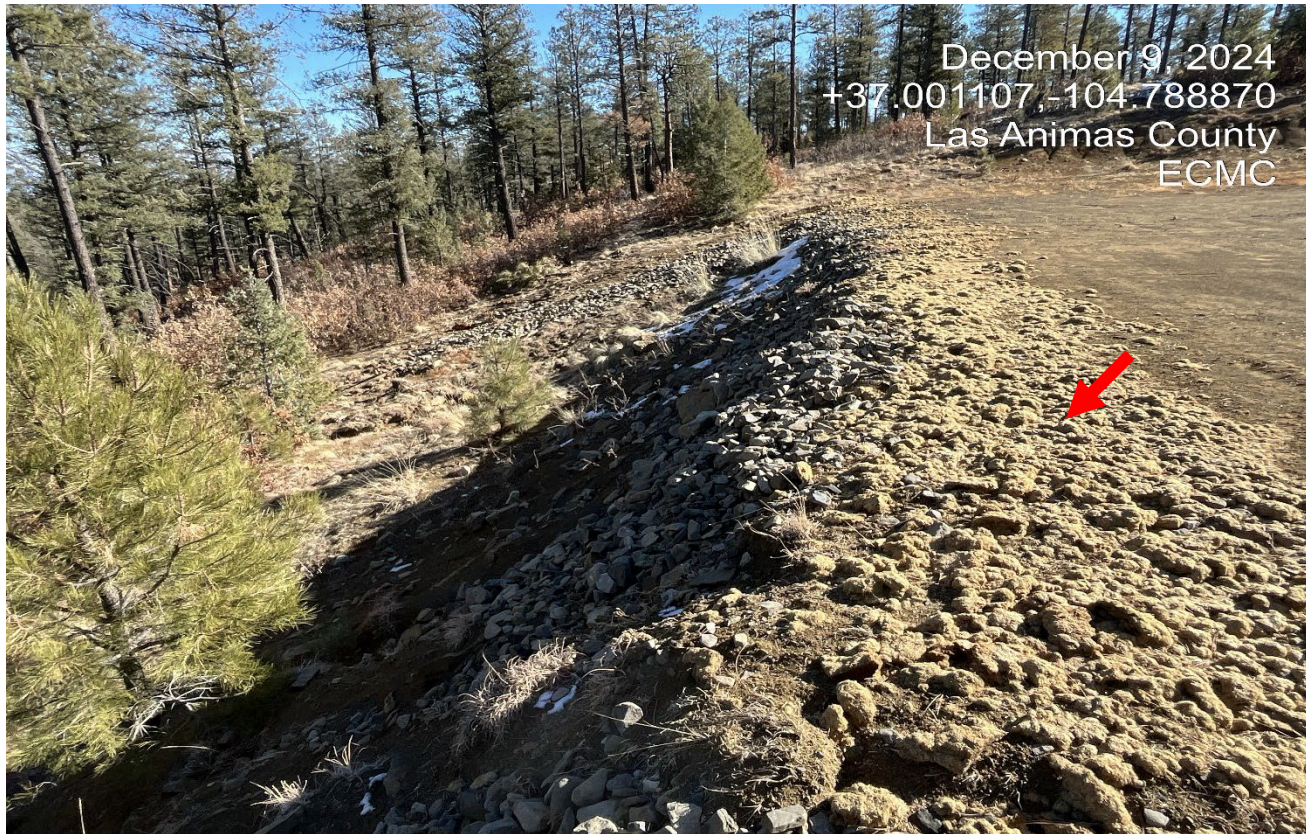
Photo 3. The fill slope was filled in with rock and some hydromulch was spread along area of the red arrow.
