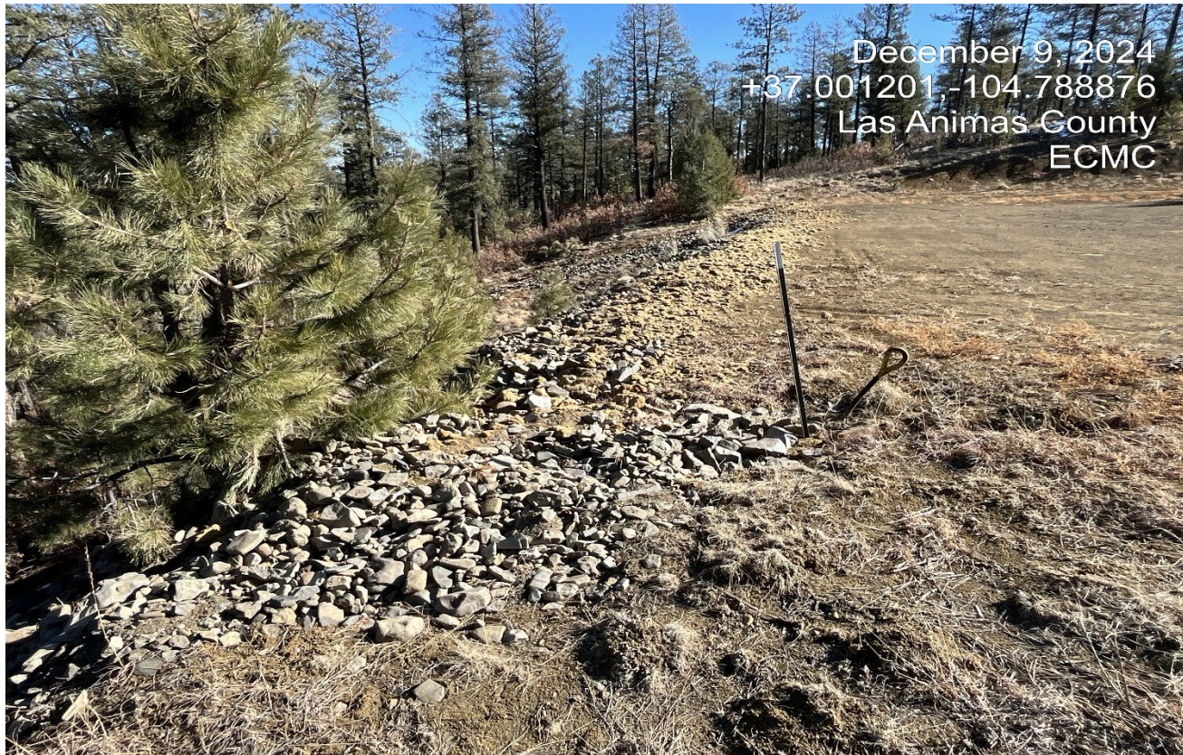
Photo 2. The erosion channels along the fill slope have been filled in with rock.
