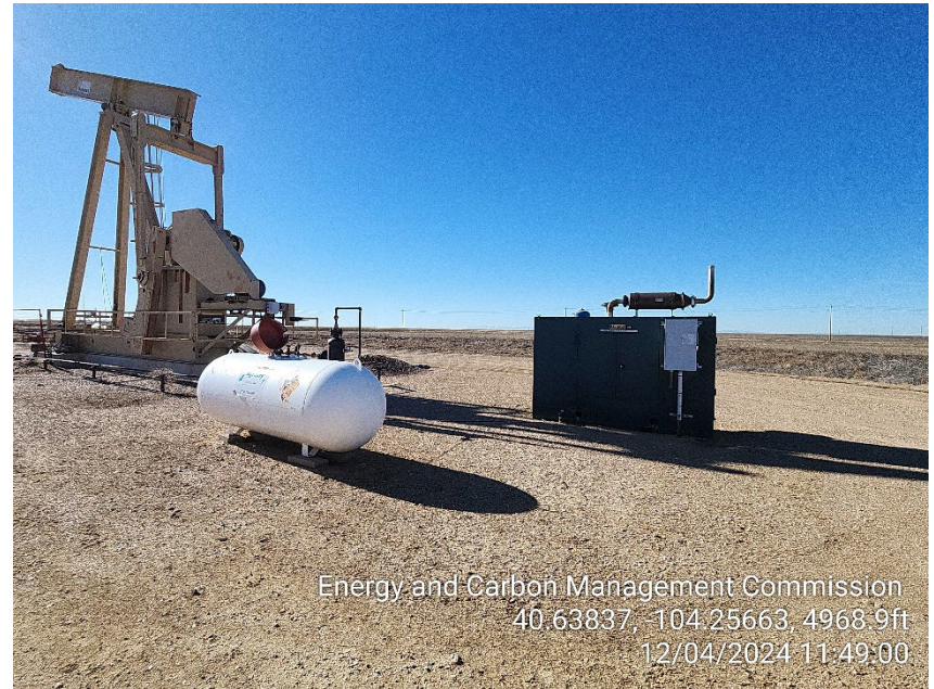
Photo 6 – Pumping Unit, Generator and Propane Tank
