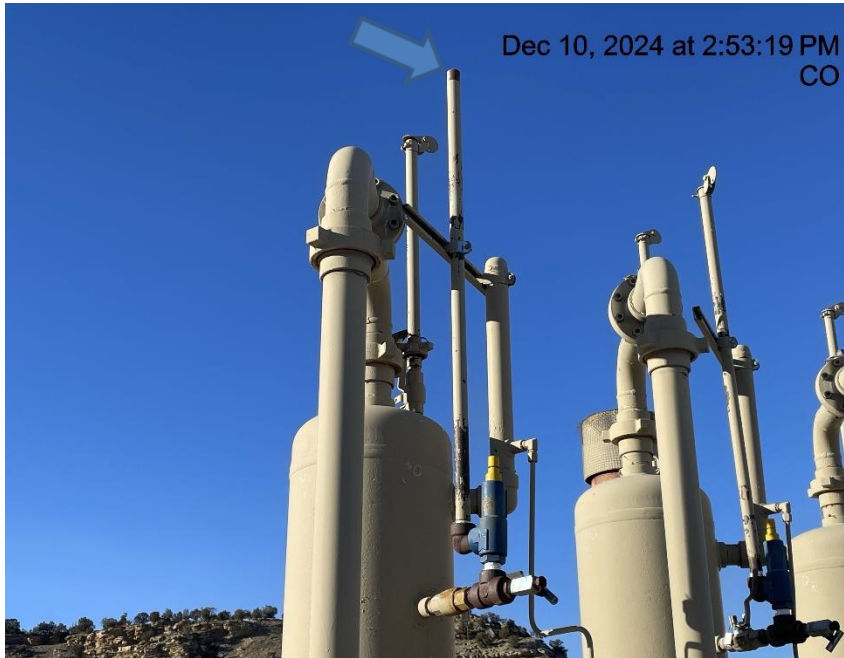
Photo # 2910 PRV vent line does not comply with CECMC pressure safety device rules
