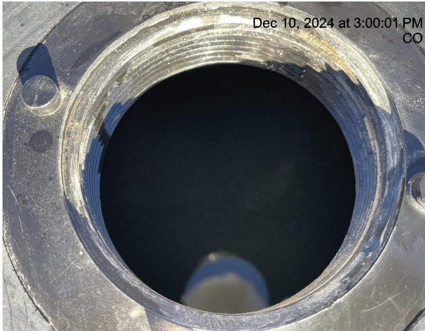
Photo # 2912 Failure to maintain chemical BMP/chemical tank containment approximately 2/3 rd full of fluid/BMP insufficient to contain possible spill
