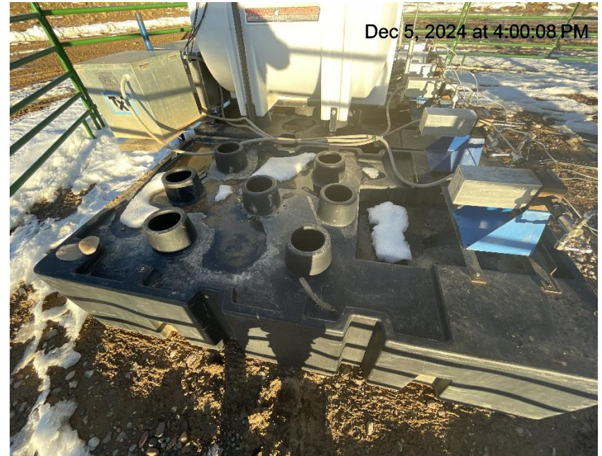
Photo # 2420 Multiple openings on chemical tank containment/available for entry by wildlife/wildlife hazard
