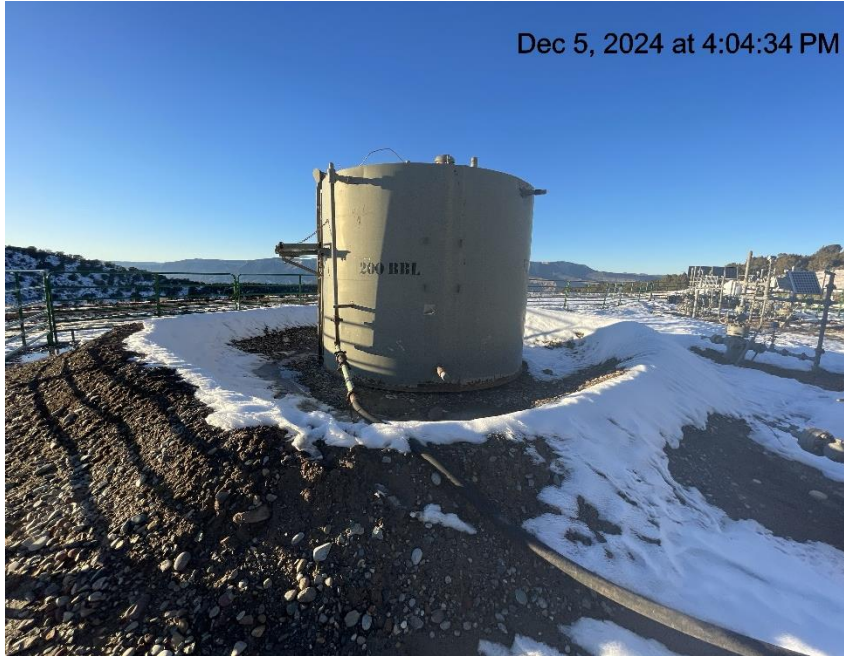
Photo # 2421 Secondary containment insufficient/does not comply with CECMC rules.
