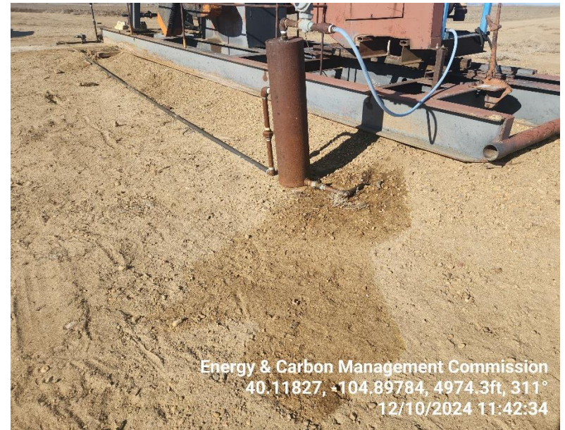
Photo 6 Stained soil by the gas engine pressure tank.
