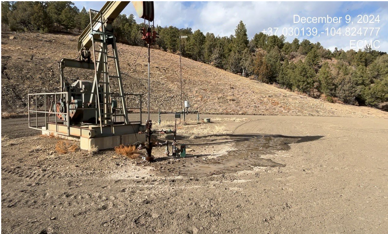
Photo 3. Facing toward the wellsite. There is a dripping water leak at the wellhead that needs to be controlled.
