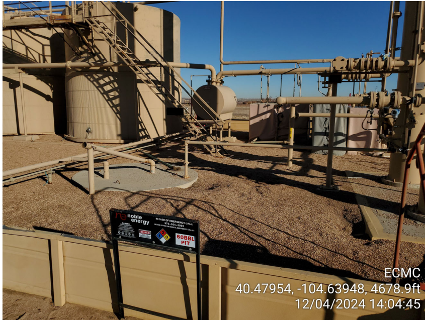
Photo 3: Buried produced water vessel and ancillary piping
