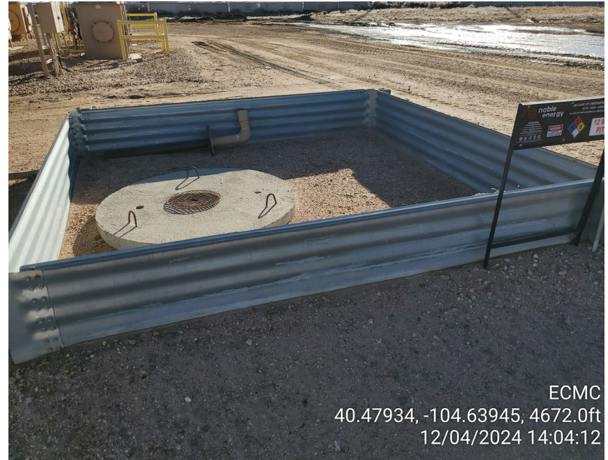
Photo 2: Partially buried vault/condensate drain near compressor
