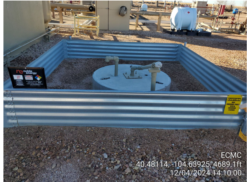
Photo 8: Concrete buried vessel near LACT
