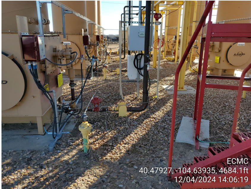
Photo 7: Process piping examples: stub ups near Emission Control Devices
