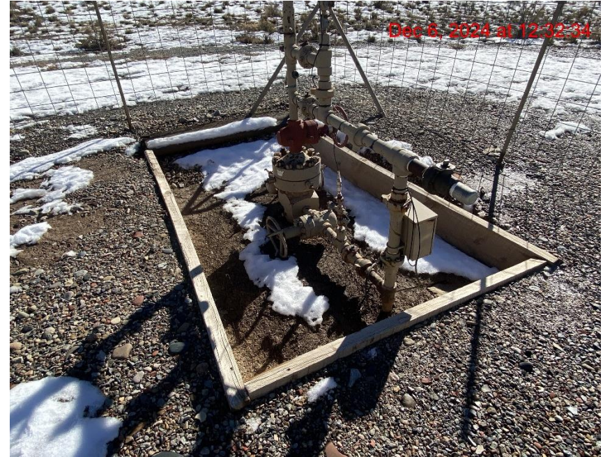
Open Wellhead Cellar/No Wildlife Egress – Photo #05202
