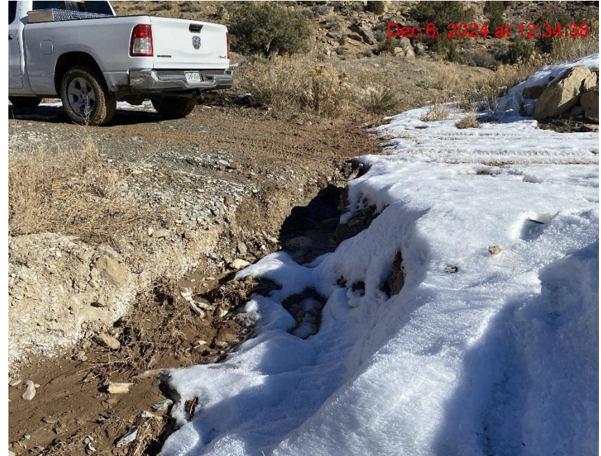
Insufficient Erosion Control/Degradation – Photo #05206
