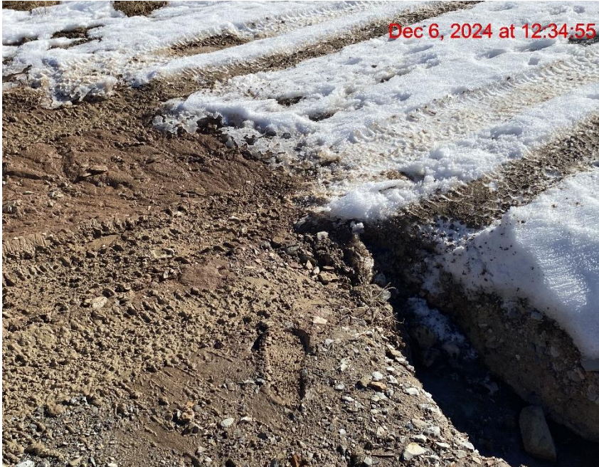
Insufficient Erosion Control/Degradation – Photo #05207
