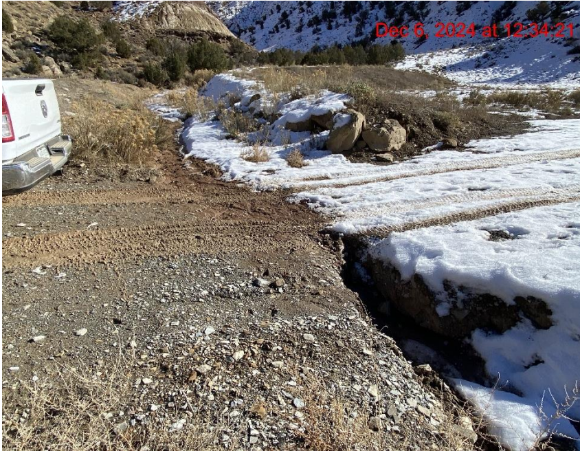
Insufficient Erosion Control/Degradation – Photo #05205
