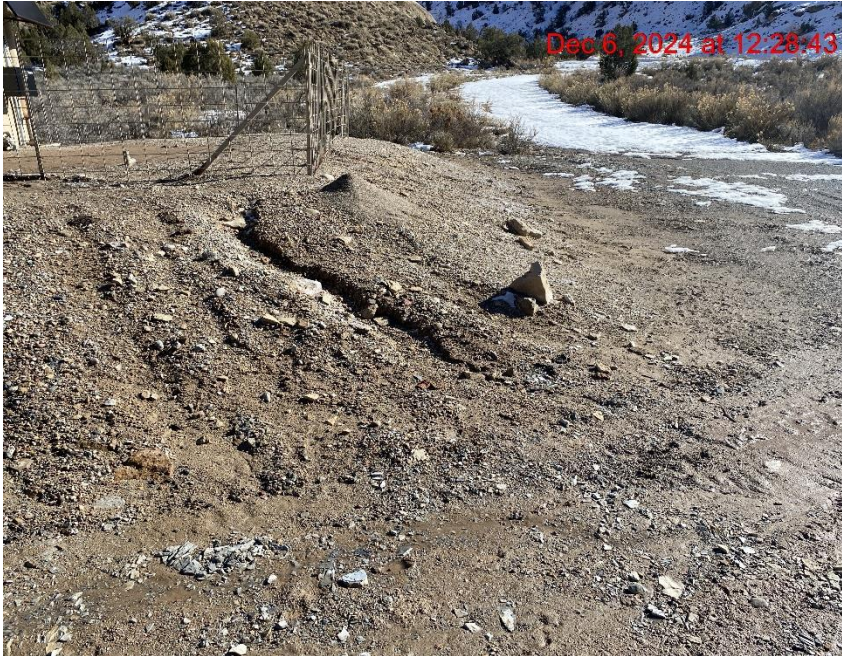
Insufficient Erosion Control – Photo #05195
