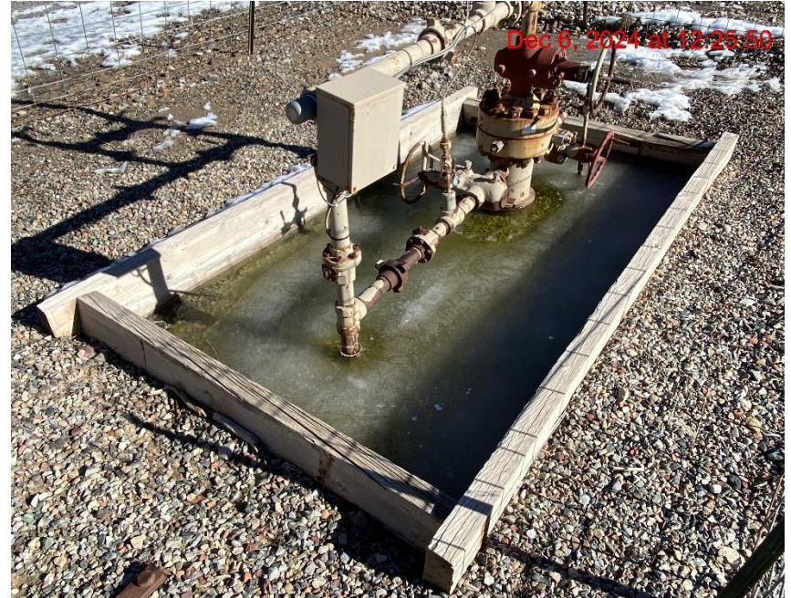
Open Wellhead Cellar/No Wildlife Egress – Photo #05191
