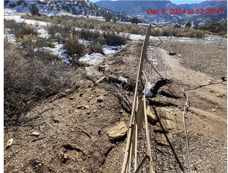
Sediment Transport Off Site – Photo #05198
