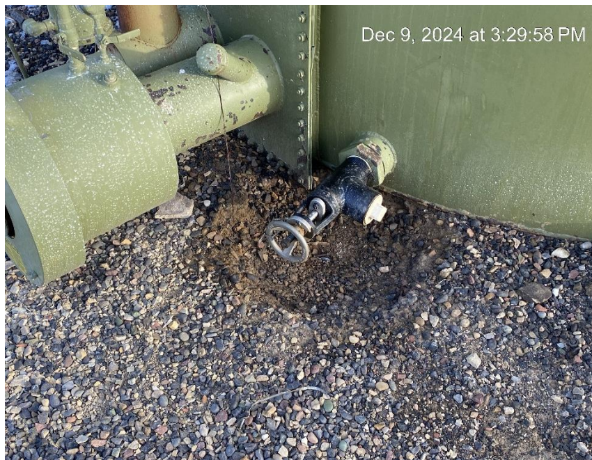
Stained soil at and around condensate tank
