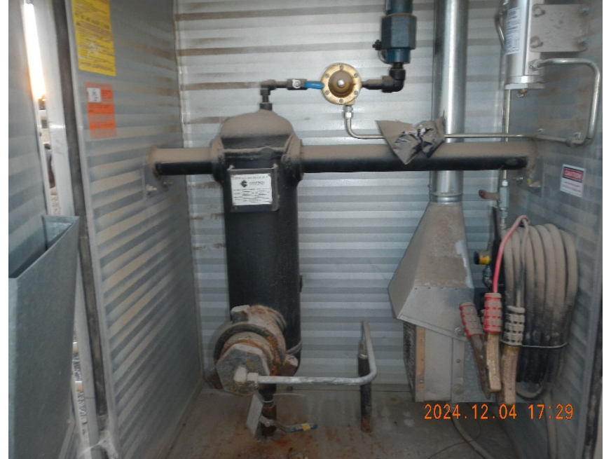
8. Vertical separator inside cabinet.
