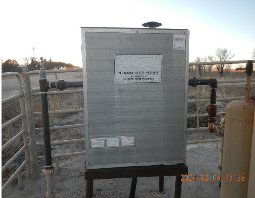
7. Flowline mounted separator cabinet at remote gathering location.
