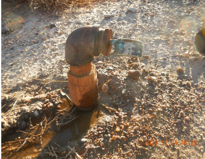
3. View of gauge that is leaking.
