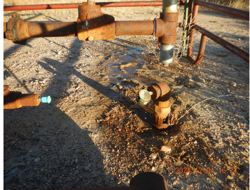
2. View of release at water line.
