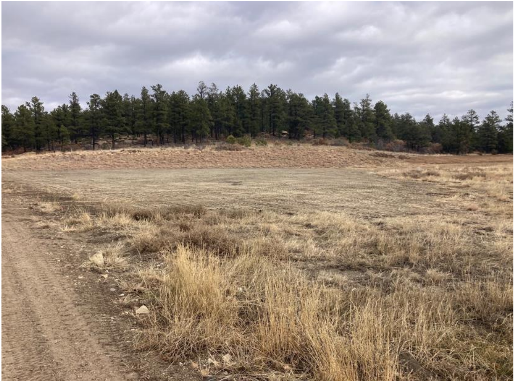
PHOTO 1: THE TWO TOP SOIL PILES HAVE BEEN SPREAD BACK INTO THE LOCATION, ALL DISTURBED AREAS HAVE BEEN TRACKED AND SEEDED TO PROMOTE VEGETATIVE STABILIZATION. THIS LOCATION WILL BE PLUGGED AND ABANDONED SPRING 2025. A FORM 6A WAS FILED FOR THIS LOCATION ON 12/04/2024.
