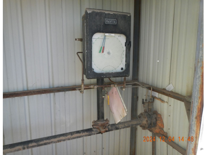
6. Shared gas meter inside shed.
