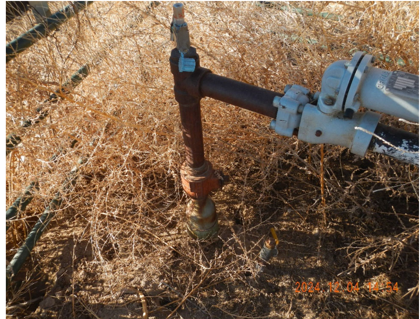
2. View of wellhead. Note dried vegetation.
