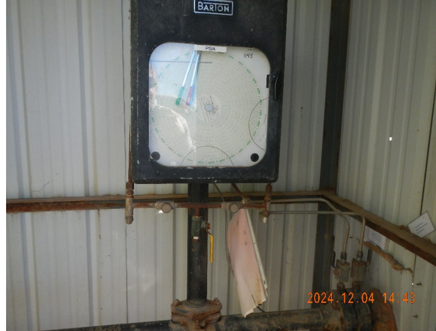
6. Shared gas meter inside shed.
