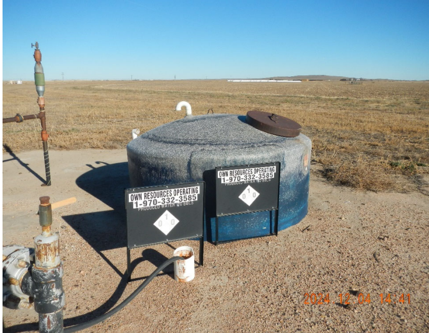
7. Produced water tanks at remote gathering location. Note faded signs.
