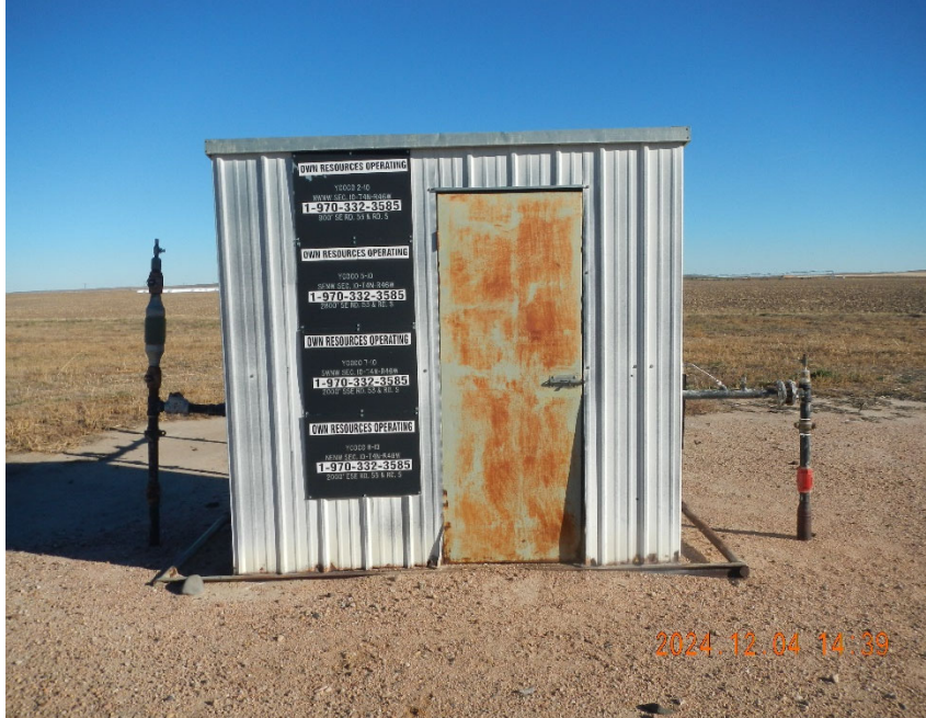
5. Shared equipment shed at remote gathering location.
