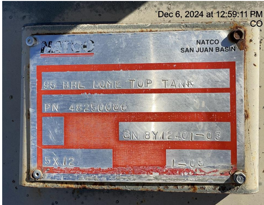
Photo # 2575 Correct tank capacity
