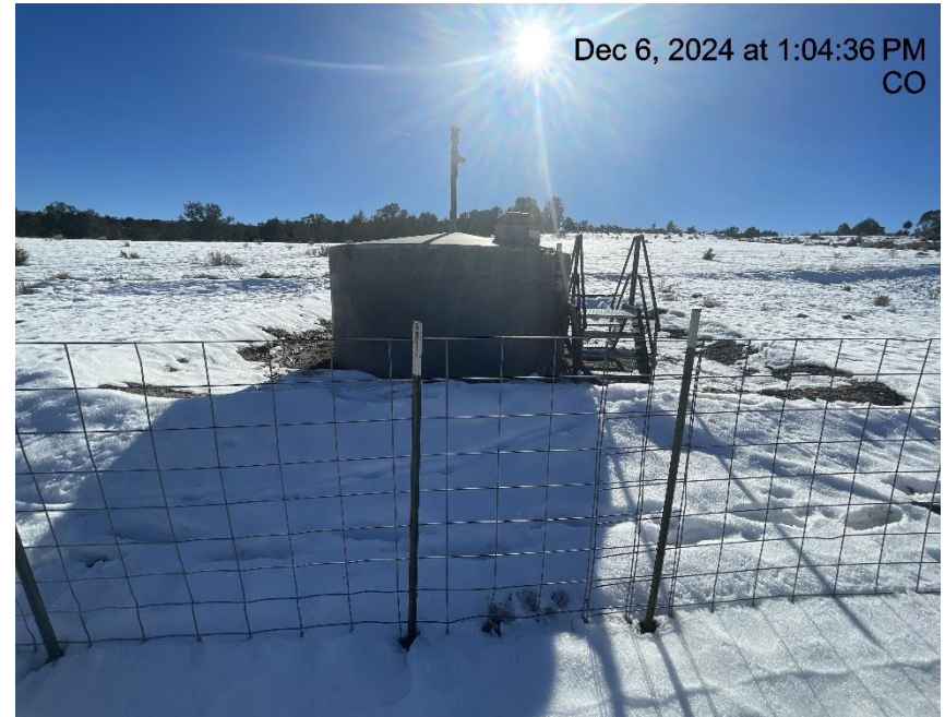
Photo # 2576 Secondary containment insufficient/does not comply with CECMC rules
