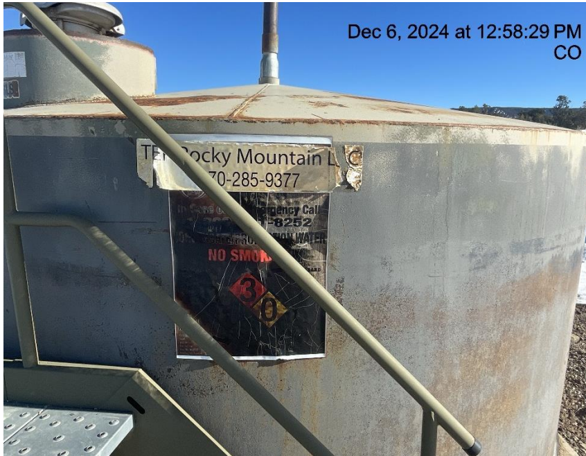
Photo # 2573 Blowdown tank label weathered & illegible /does not comply with CECMC rules. Additionally capacity on tank label is also incorrect
