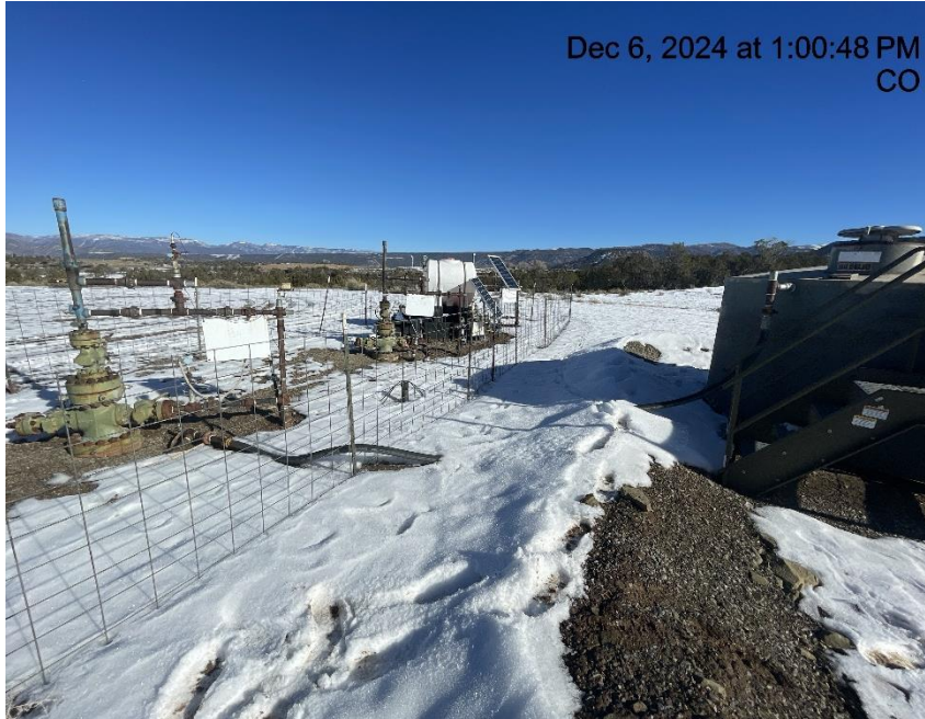
Photo # 2581 CIRCLE B LAND 14C-35-692 well bradenhead line connected to blowdown tank
