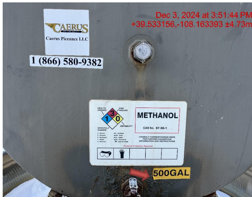
Photo # 0269 Capacity label is peeling on methanol tank
