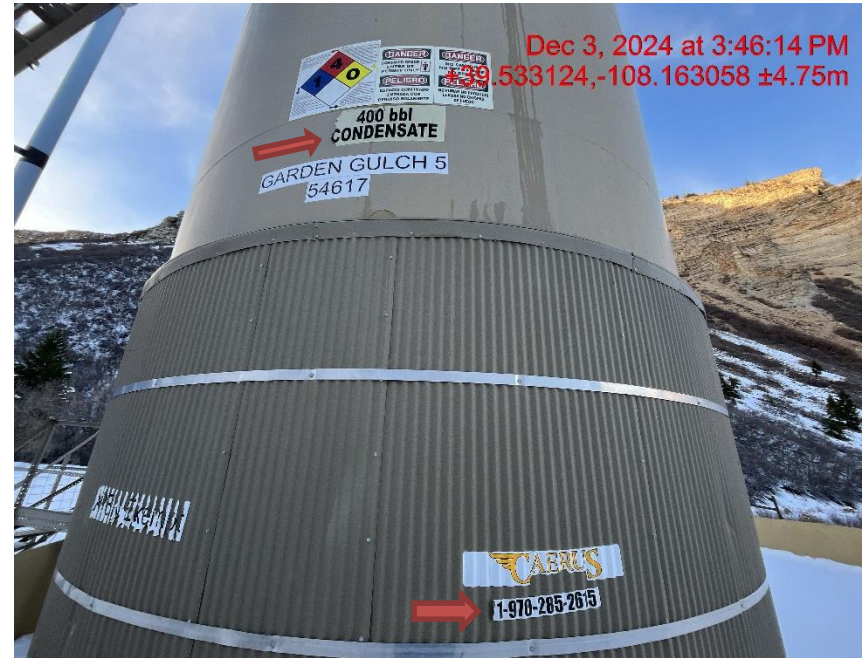
Photo # 0257 Some information on condensate tank is peeling
