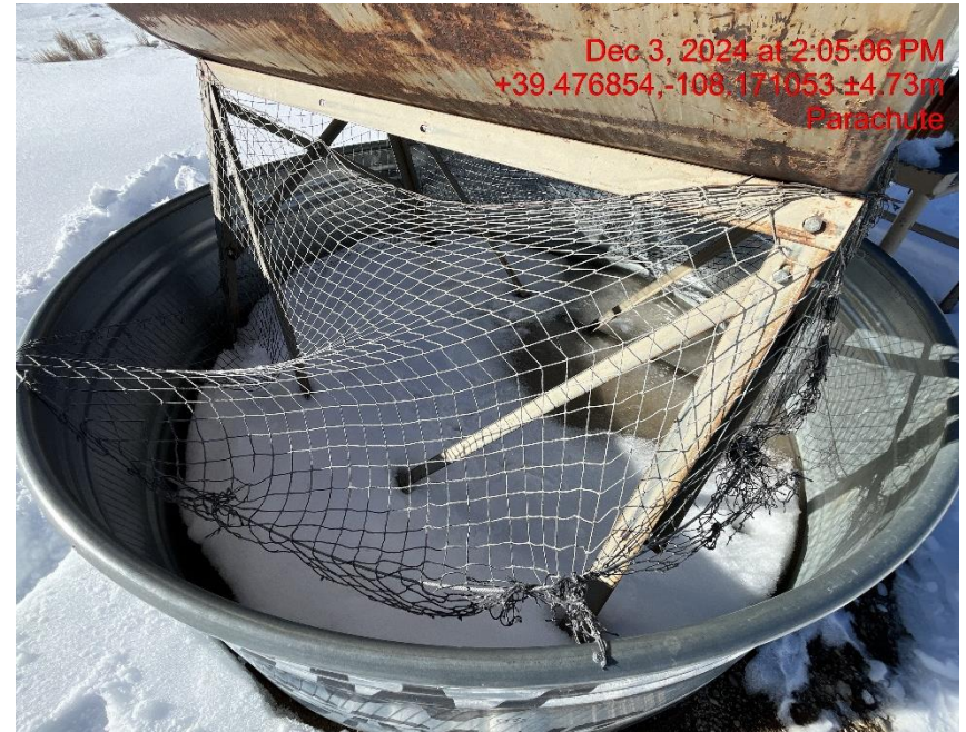
Photo # 0209 Wildlife protection for Methanol tank containment needs maintenance/netting is damaged and open to wildlife
