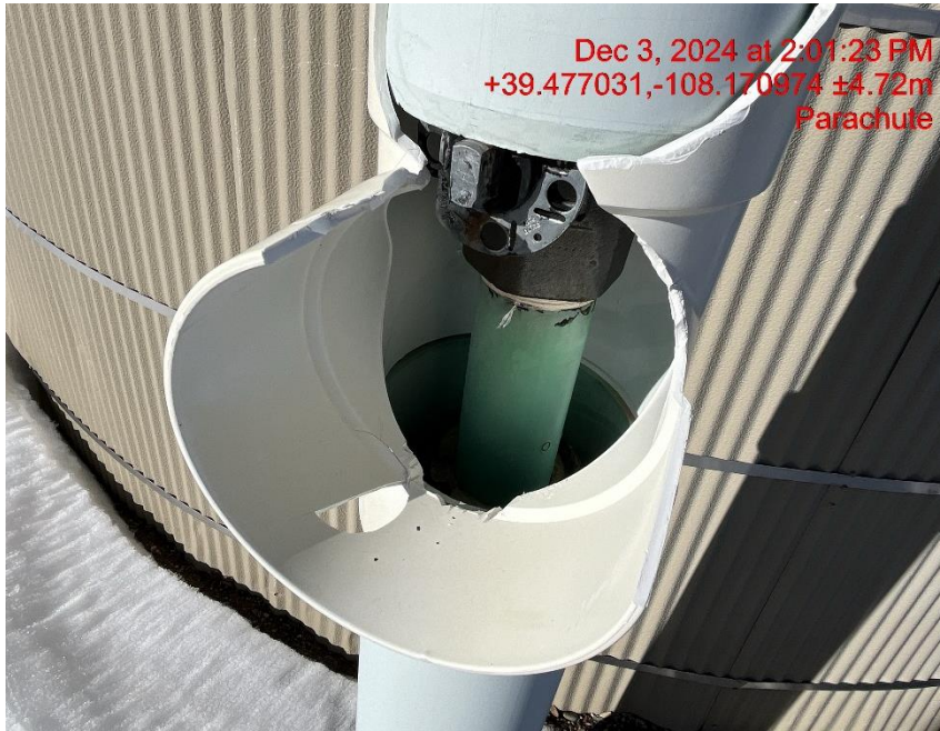
Photo # 0203 Flow line heating insulation open ended/wildlife hazard available for entry by wildlife
