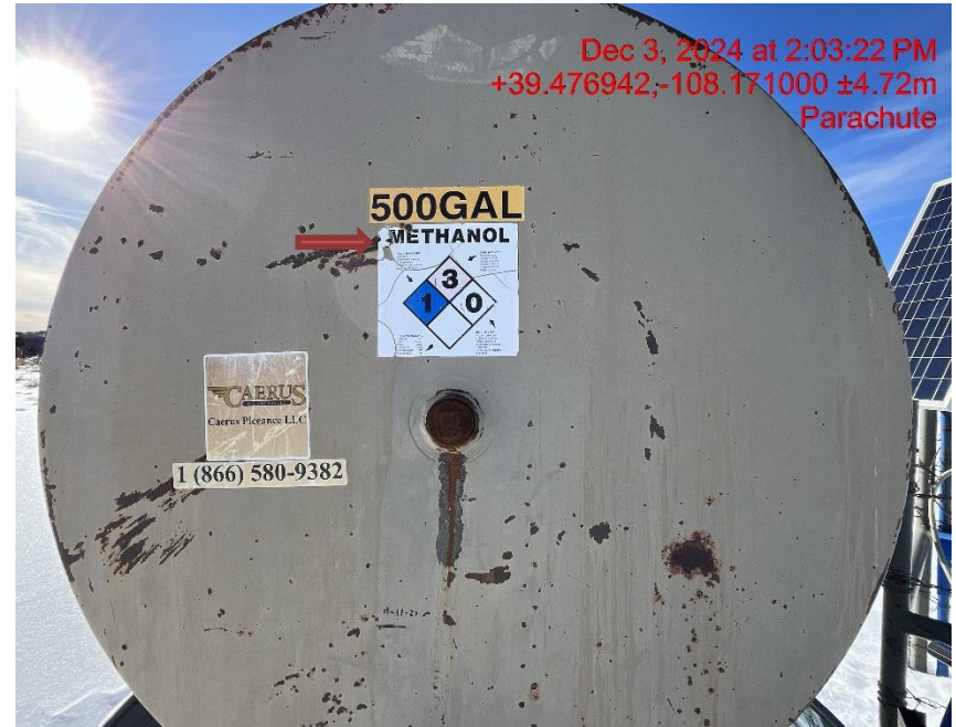
Photo # 0206 Some information on methanol tank is peeling and becoming illegible
